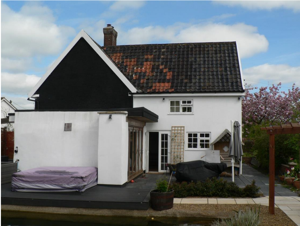
Figure 7. View showing the existing garden room wall where new window openings are proposed
