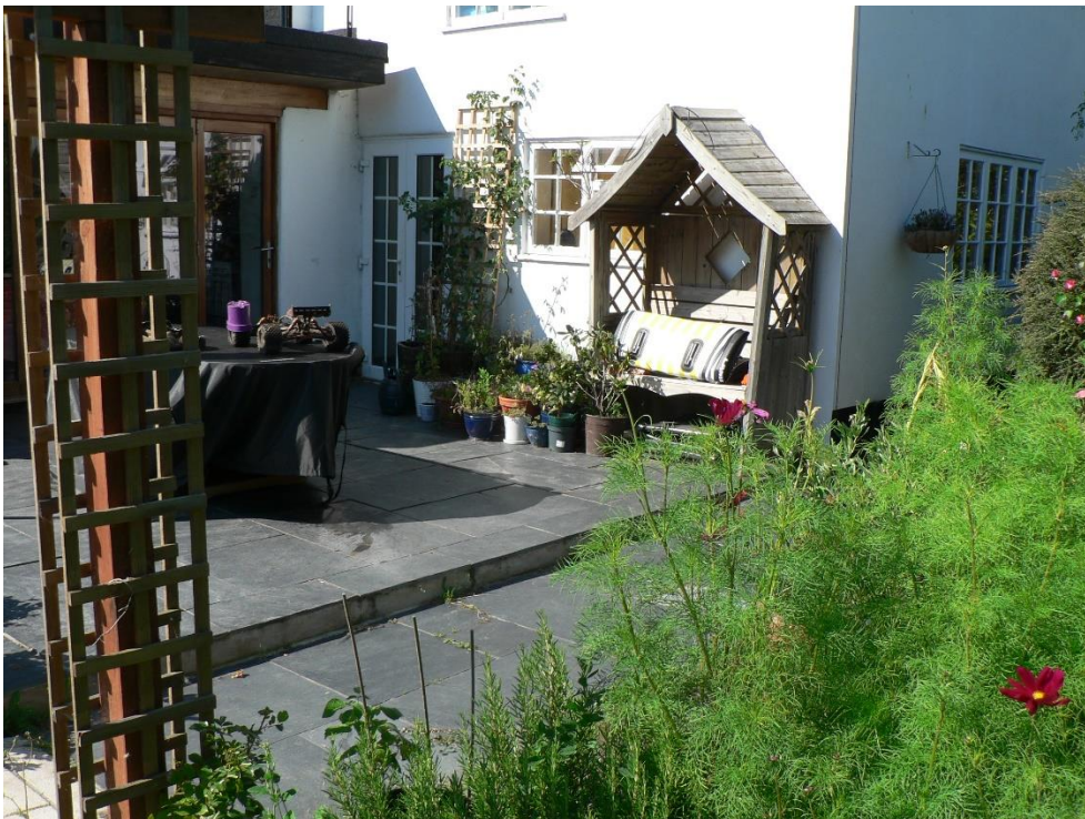
Figure 9. View showing the existing dining area external wall where the proposed bi-fold door opening is proposed
