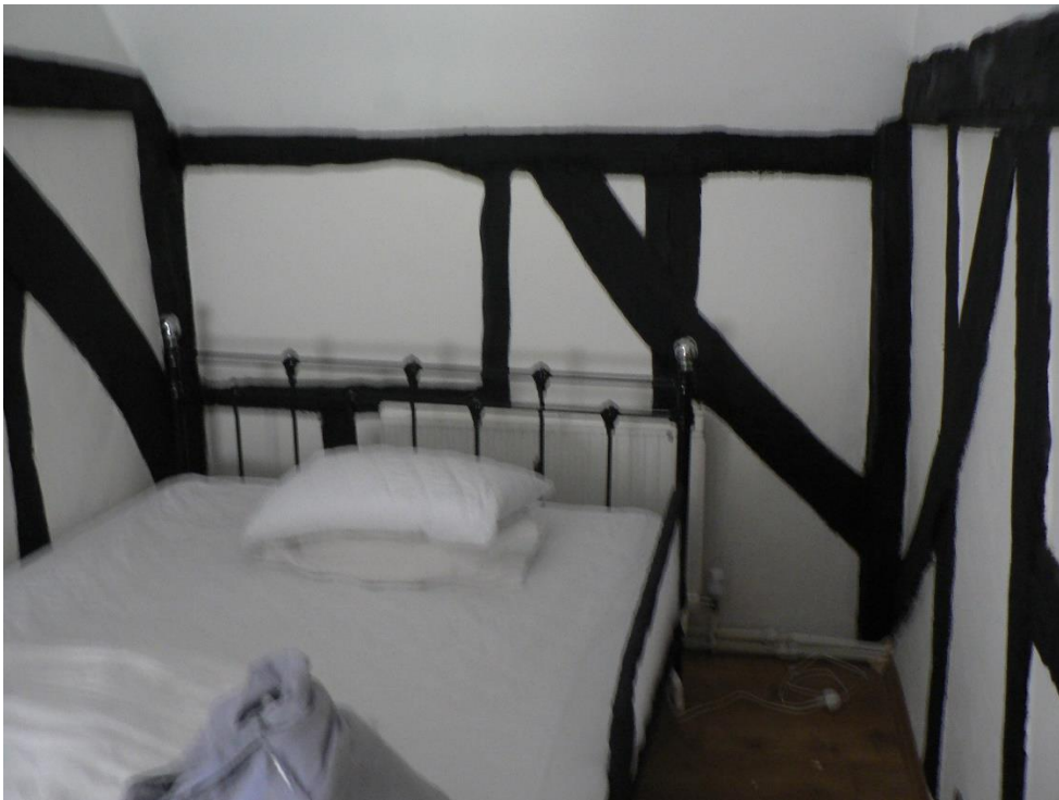
Figure 5. View showing the existing landing area to be the new first floor shower room
