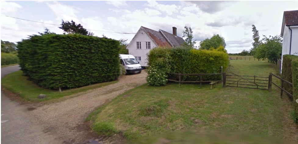
Figure 2. South facing view of Greenways Farm from the vehicular site access off Flaxlands
