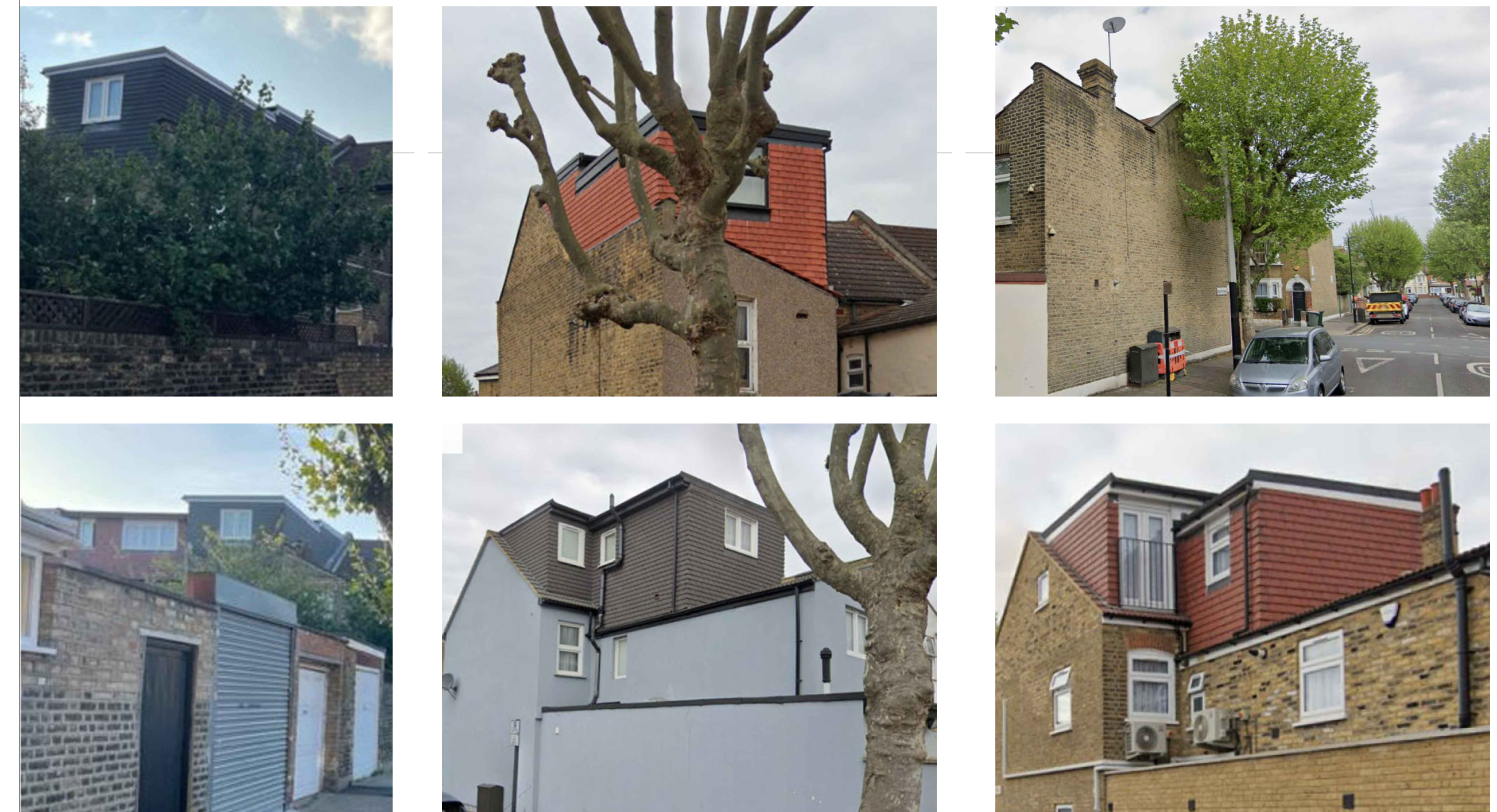
End of terrace example dormer extension in and around the proposed site
