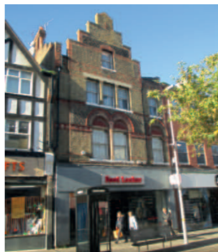
161 High Street Year: 1890-1898 Style: Tudor Revival Materials: London Stock brick Windows: Sash Flemish style influences,
