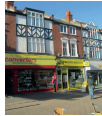
189 to 199 High Street Year: (unknown) Style: Regency-Tudor Style Materials: Stock brick with hipped slate roof and terracotta ridge tiles Windows: French
