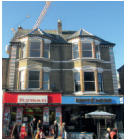
119 to 121 High Street Year: 1866-1880 Style: Gothic revival Materials: Stock brick with red brick banding detail, slate roof and three-hole crested ridge tiles Windows: sash
