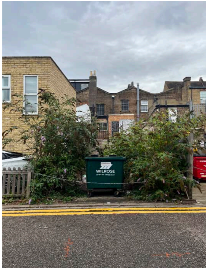
212 High Street- Rear Elevation
