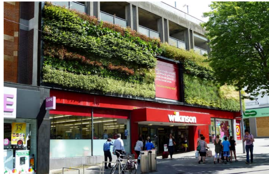
Trinity Square looking East
