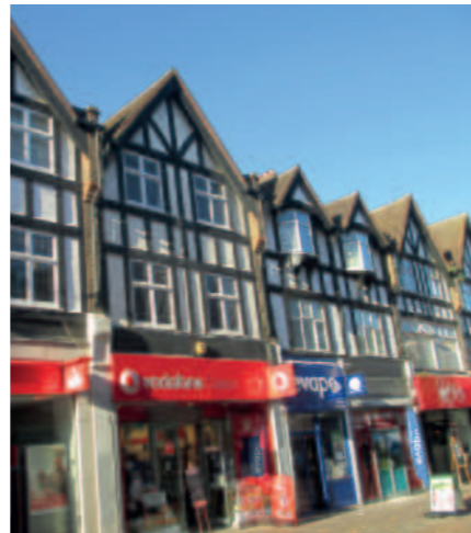
151-159 High Street Year: 1924 Style: Tudor Revival Materials: Red Stock brick Windows: uPVC Distinctive Gables with studs and braces
