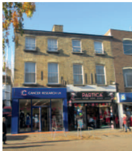
123 to 125 High Street Year: 1866-1895 Style: Classical Revival Materials: Stock brick with hipped slate roof and terracotta ridge tiles Windows: Sash
