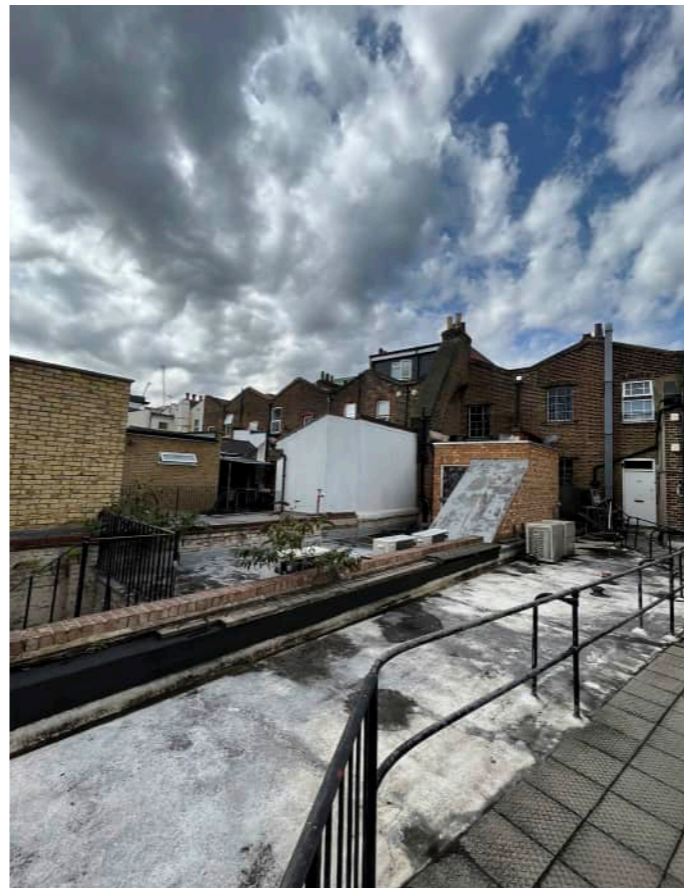
212 High Street - Rear Exterior View
