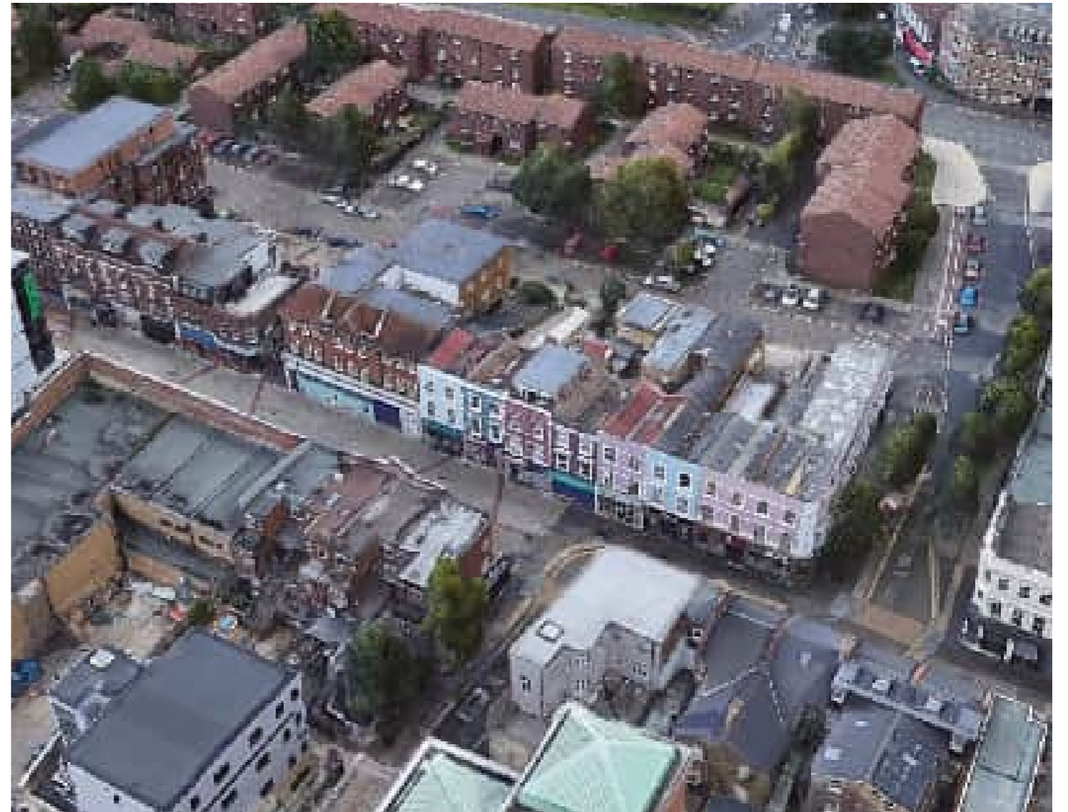
212 High Street- Aerial View
