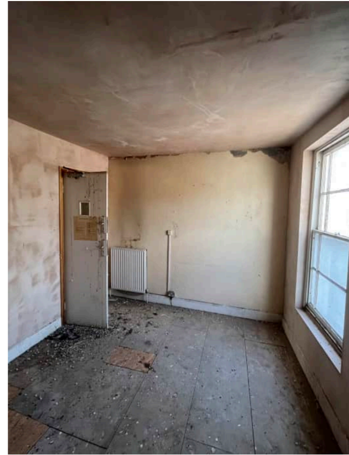
212 High Street- First Floor Space
