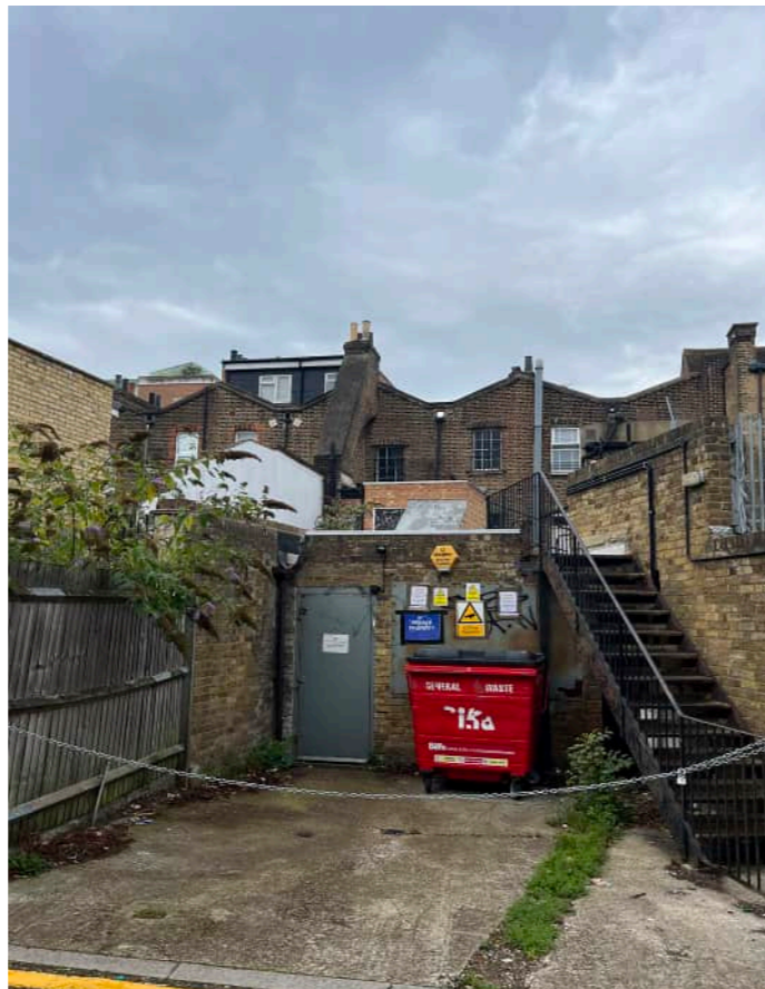
212 High Street- Rear Exterior Access
