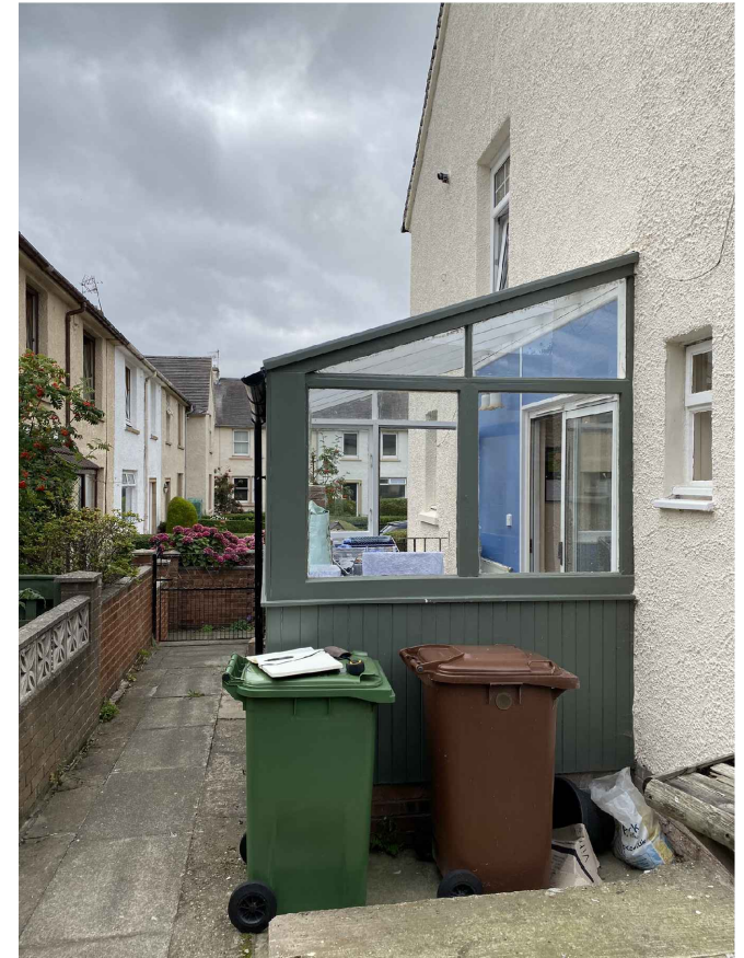
Existing lean-to rear elevation
