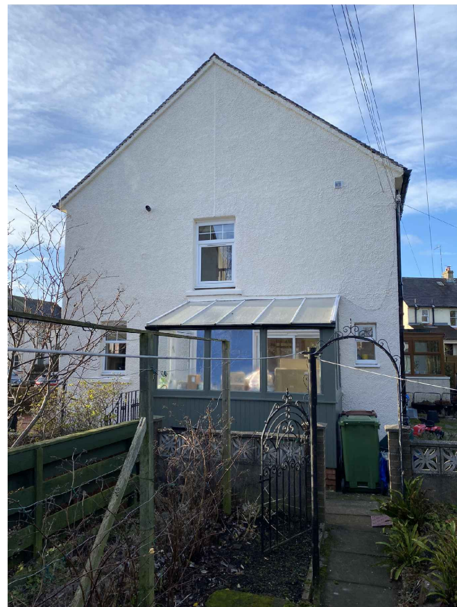
Existing house side elevation from garden plot
