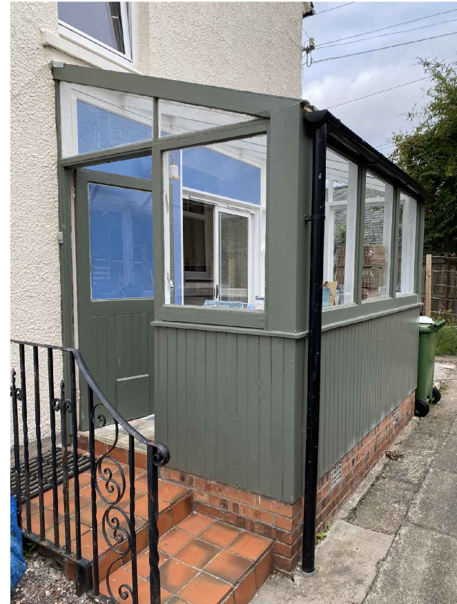
Existing lean-to oblique view from shared access path
