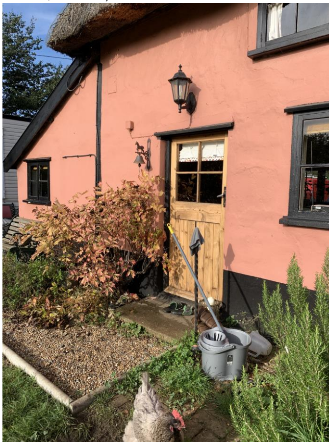
Plate 2: Location of proposed new porch at back door of Brome Cottage (Photo: O. Robson, 30/10/23)
