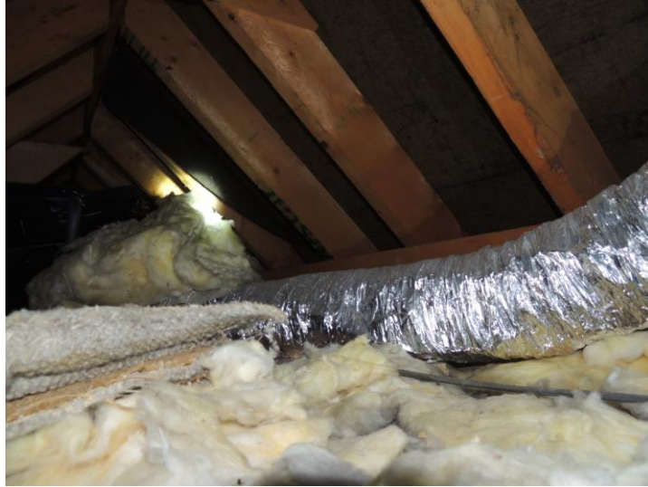
Photo 9: Note lack of evidence of bats on floor of loft
