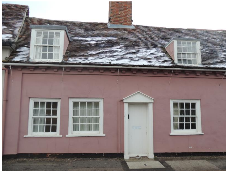
Photo 2: Front (western) elevation. Note dormer windows
