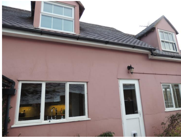
Photo 6: Southern elevation of extension
