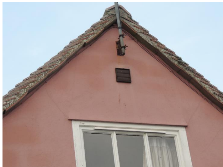
Photo 5: Note tight seal to gable
