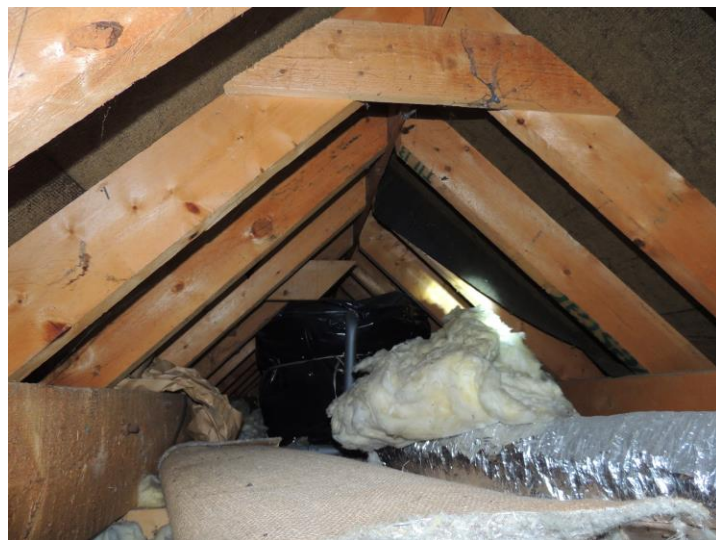
Photo 8: Note lack of evidence of bats in shallow-pitched loft
