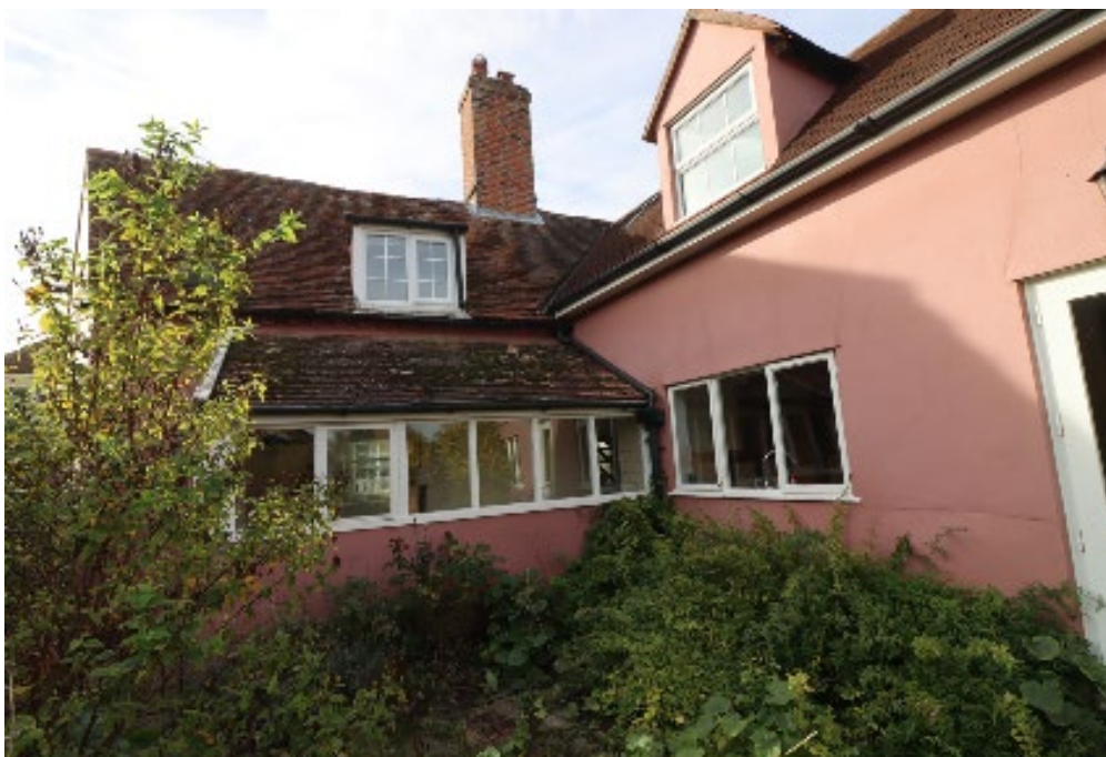
Rear view of existing cottage with C20th lean-to and C20th 1.5 storey rear wing.
