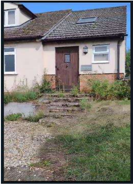
Front door & steps
