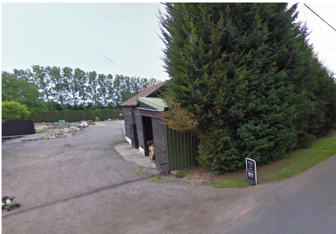
View looking into the site with building to be demolished shown to centre of image
