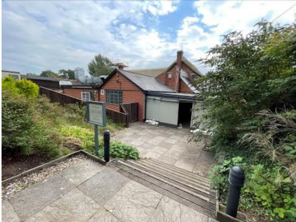
Rear view on to the rear of the property looking down from the stepped patio area
