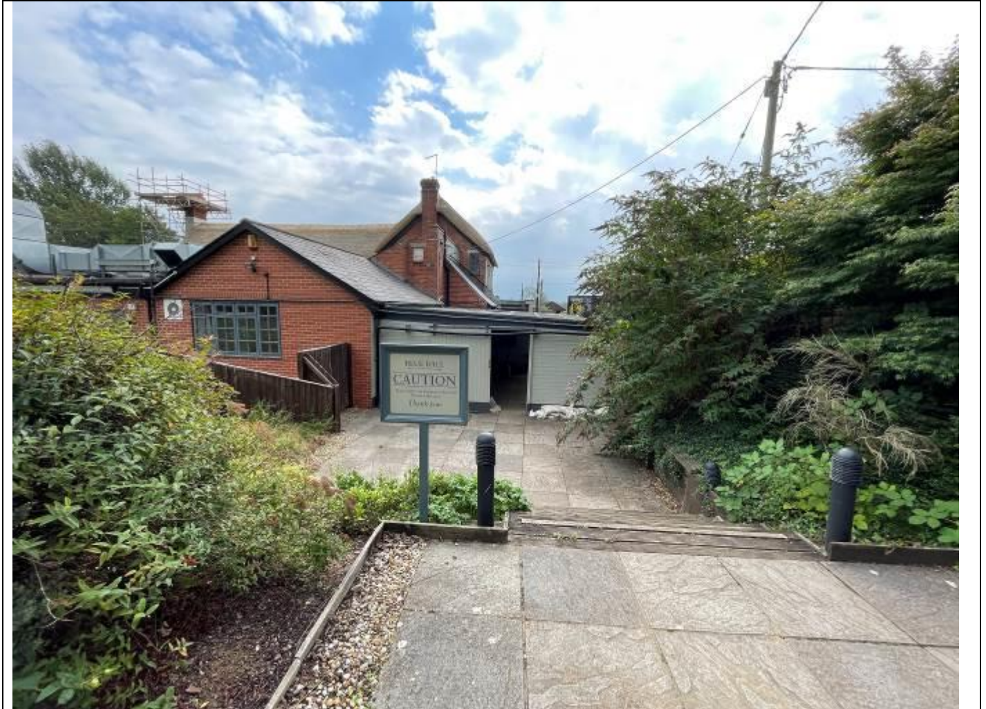
Rear elevation showing the existing covered structure
