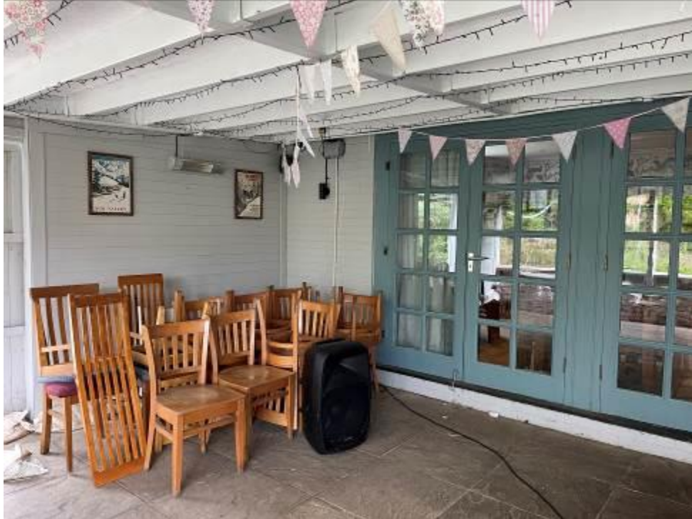
View from underneath the current flat roof extension looking back towards the access doors into the pub
