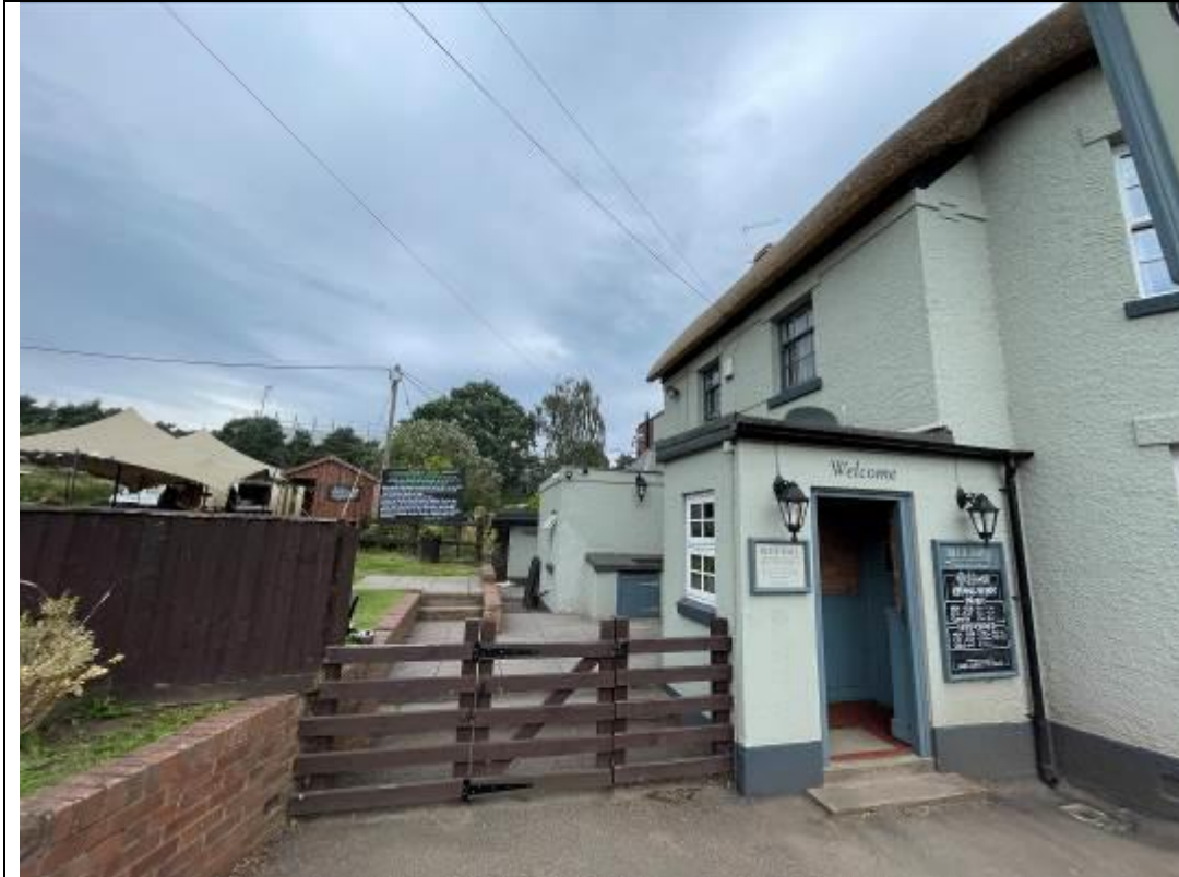
Roadside elevation looking back towards the proposed location of the extension
