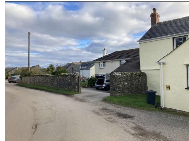
MAIN (NORTH) ELEVATION AS SEEN FROM ROAD
