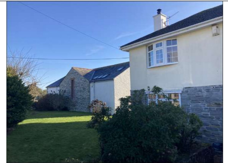
MAIN (NORTH) ELEVATION WITH ADJACENT 'THE COTTAGE' IN THE BACKGROUND
