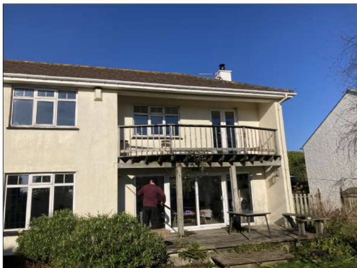
REAR (SOUTH) ELEVATION WITH BALCONY IN VIEW
