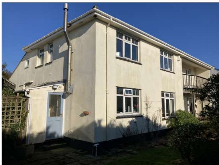
REAR AND SIDE (SOUTH AND WEST) ELEVATION WITH LEAN TO TO BE REMOVED
