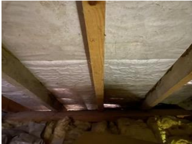
Photograph 2 – internal loft space continued. Light coming through.
