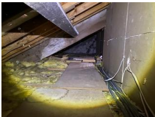
Photograph 1 – internal loft space.
