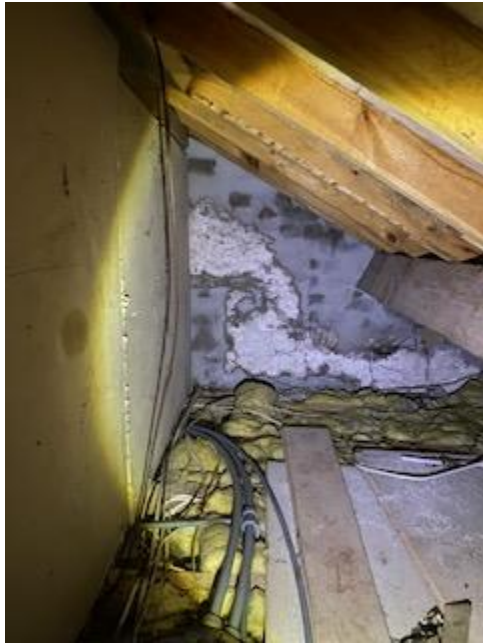
Photograph 4 – loft space continued.
