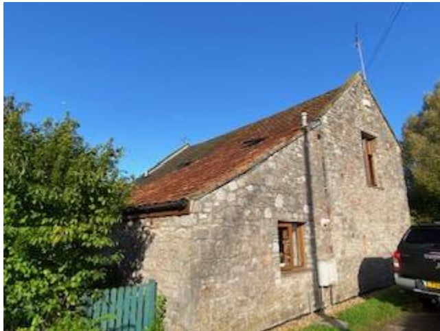
Photograph 7 – southern and eastern elevations of building.
