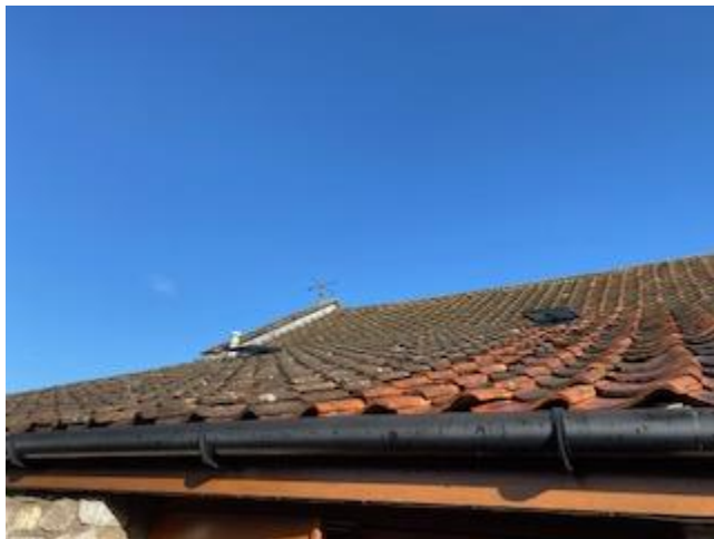
Photograph 8 – southern elevation on building.
