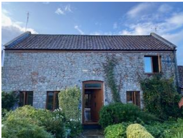
Photograph 5 – northern elevation where proposed porch way will be located.
