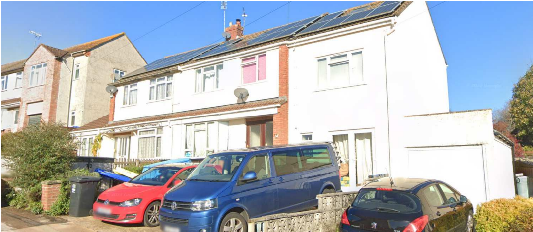
Above: Neighbouring properties nearby the application site
