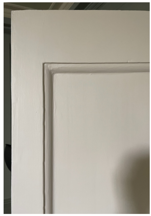
Photograph of existing door from landing
