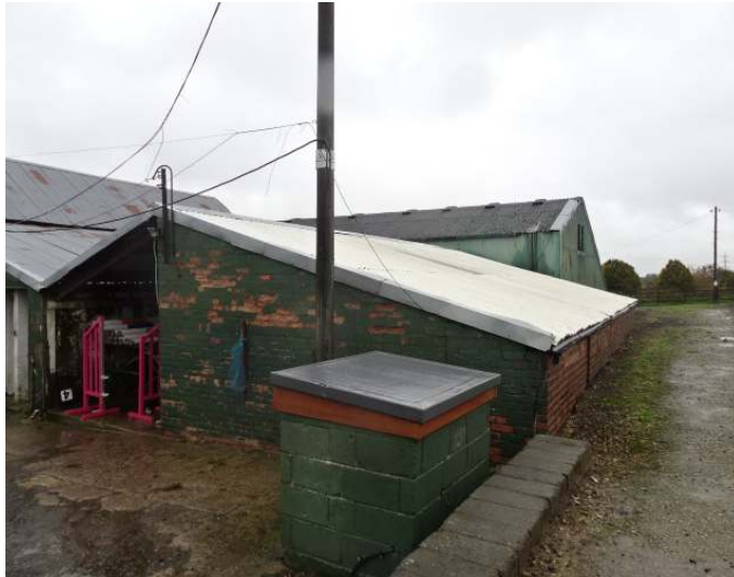
West elevation, equipment store
