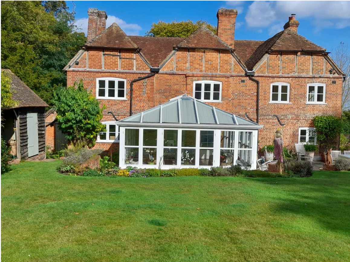
Fig. 6: View, looking north-east, of the rear south-west elevation of Church Farm House.
