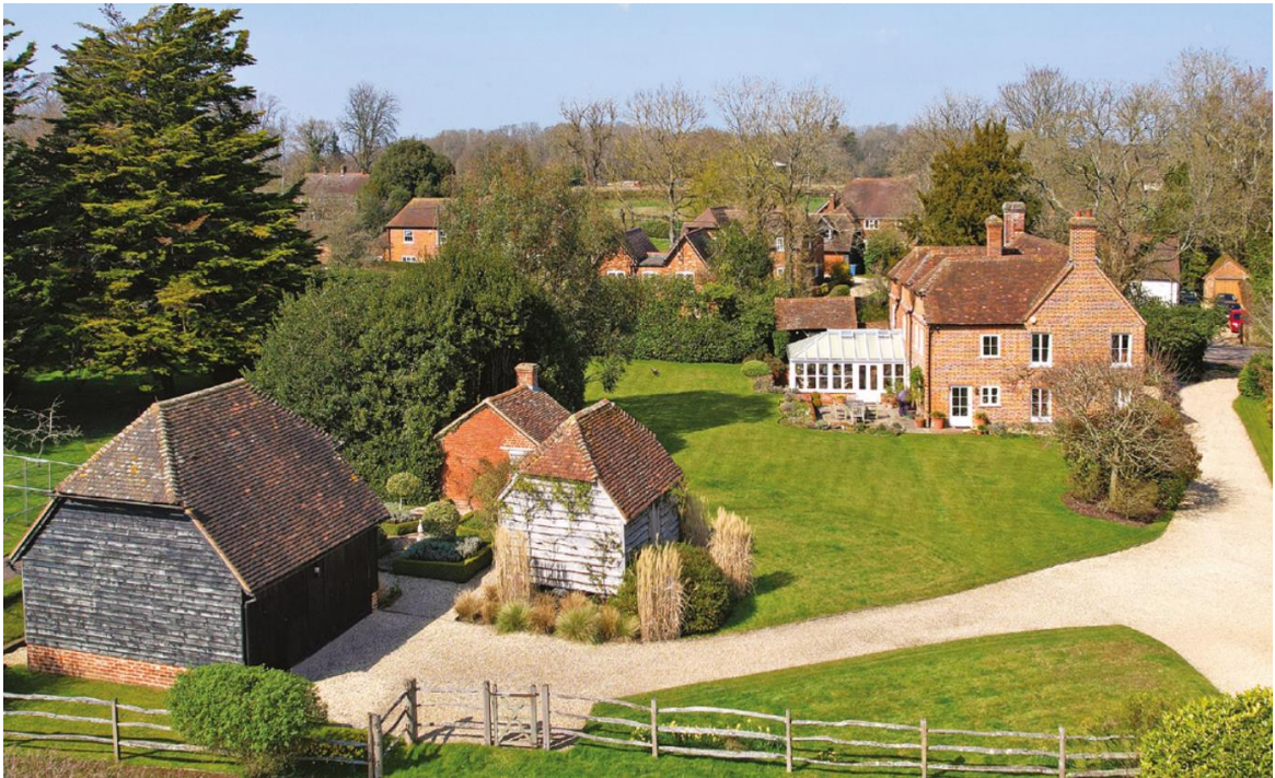
Fig. 7: View, looking north, of Church Farm House within its garden setting, including the Grade II-listed Granary and adjoining buildings to the south (Knight Frank).
