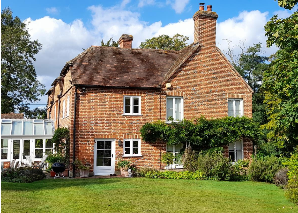
Fig. 5: View, looking north, of the south-east elevation of Church Farm House.
