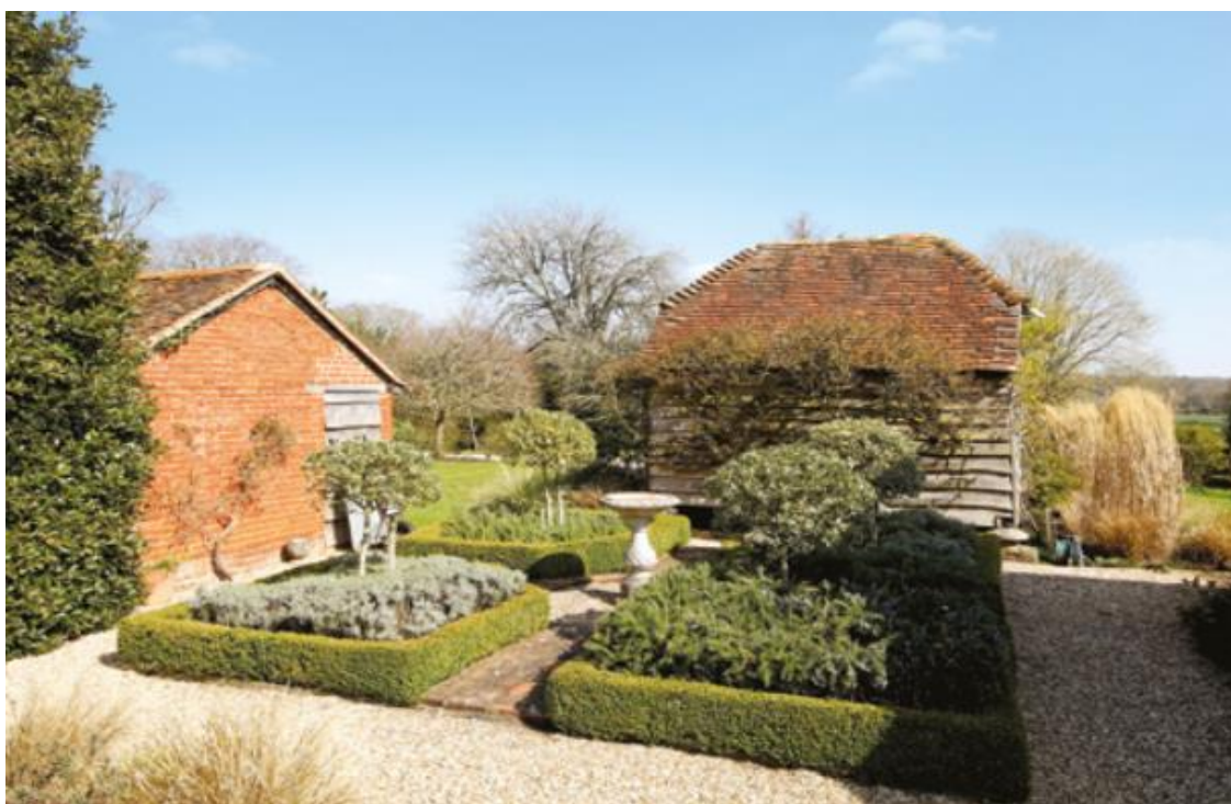
Fig. 17: View, looking west, of the Grade II-listed Granary to the south of Church Farm House (Knight Frank).
