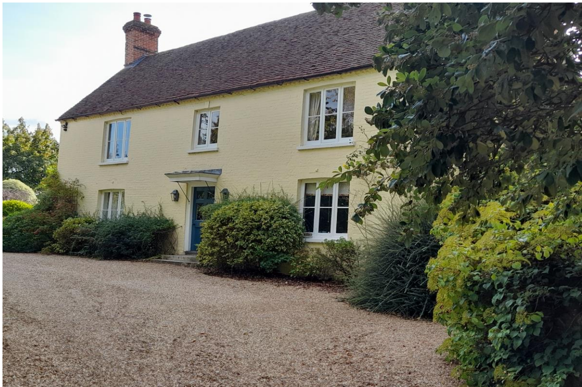
Fig. 4: View, looking south, of the north-east elevation of Church Farm House.
