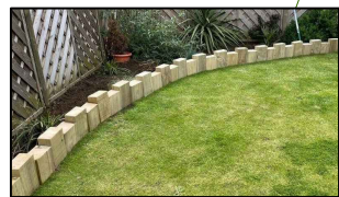
SLEEPER STEPS / LOW RETAINING WALL
