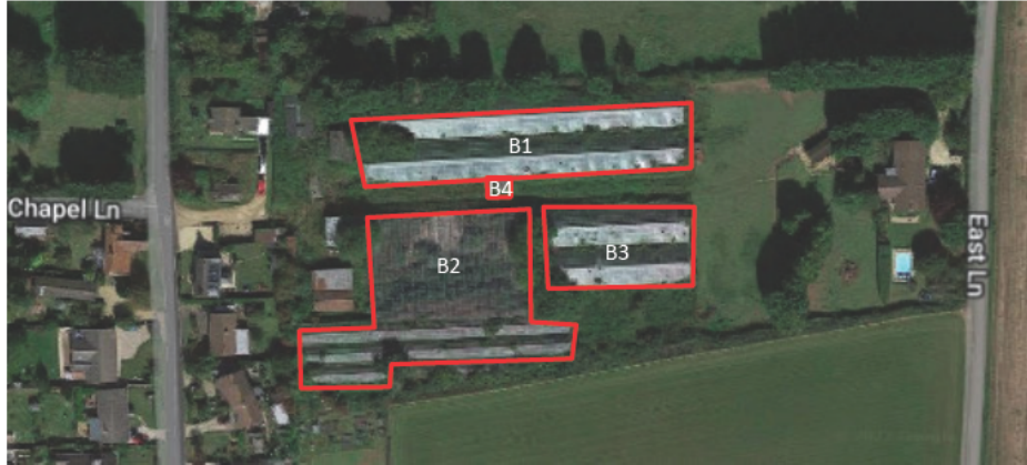
Figure 7. Location showing the buildings within the site (Google Maps, 2022)
