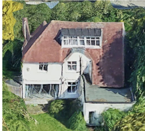
Fig. 7 – Elmwood- View facing Warboys Road
