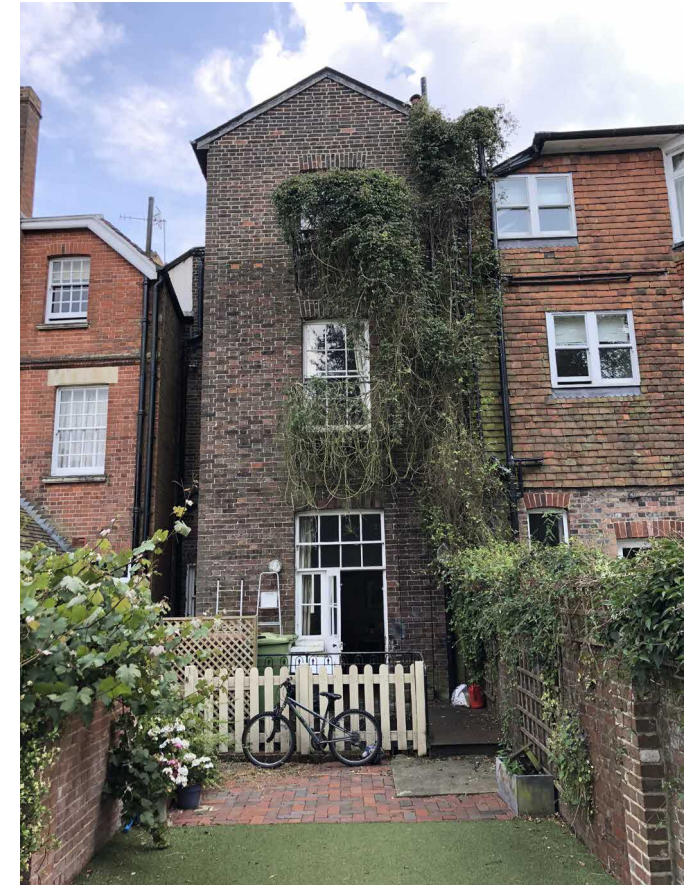
view of rear elevation and garden access
