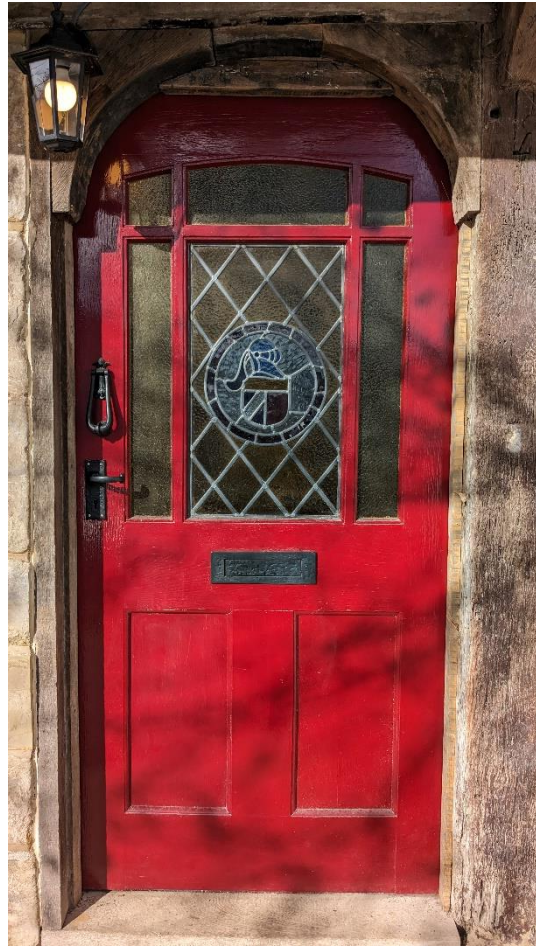
Figure 1: Approved front door details (left) and installed front door (right)
