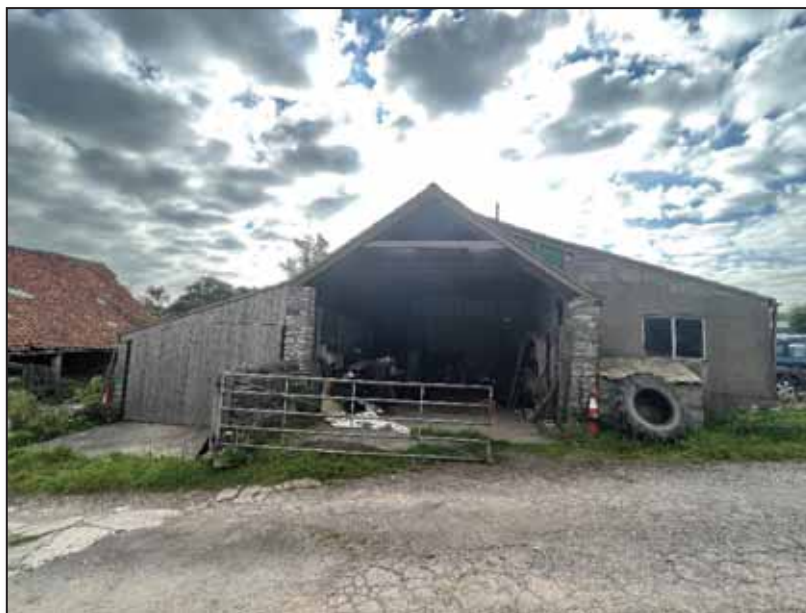
Image 13: Building 1, front southwest facing elevation
