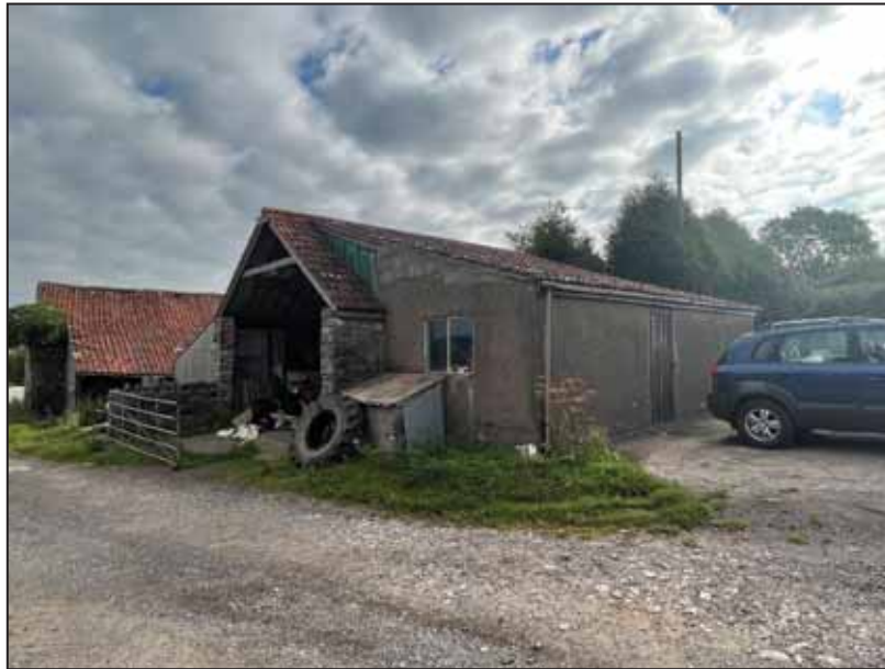
Image 14: Building 1 looking north
