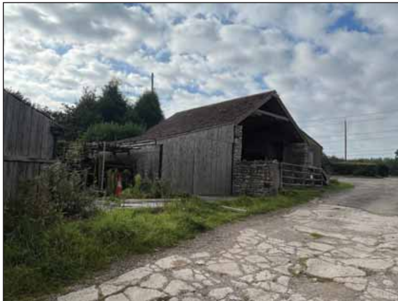
Image 15: Building 1 looking southeast
