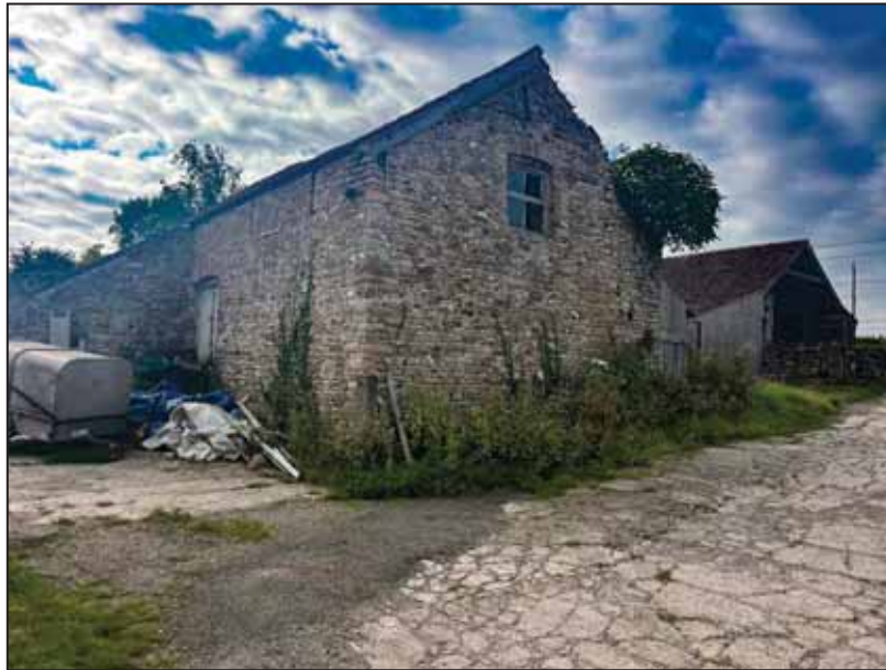
Image 17: Building 2 viewed from north
