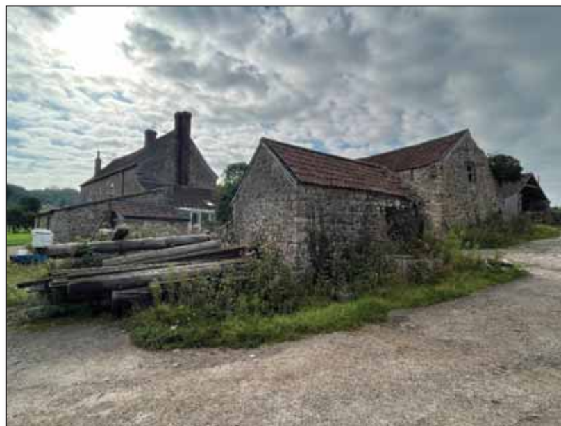
Image 4: Lower Woodhouse Farmhouse with the three outbuildings to the right
