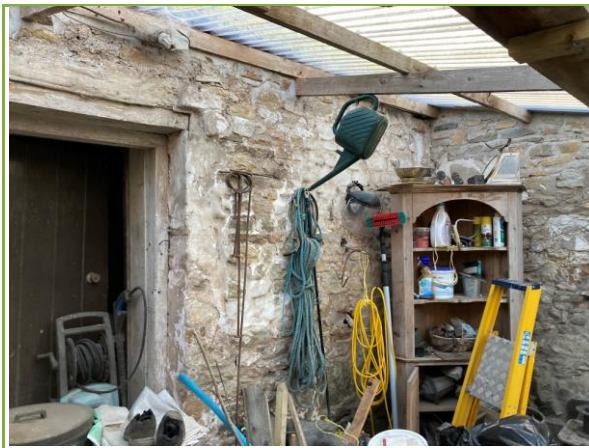
Interior (lean-to on north-eastern elevation)
