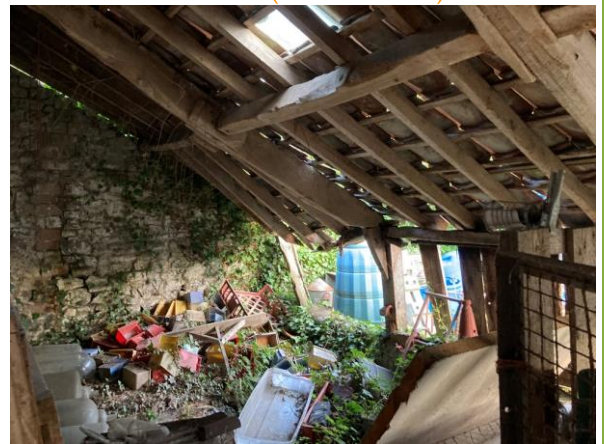
Interior (lean-to on south-western elevation)
