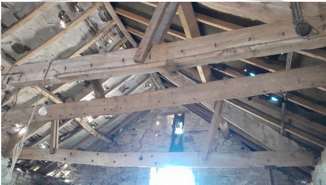
Photo 1: Central area roof internal view
