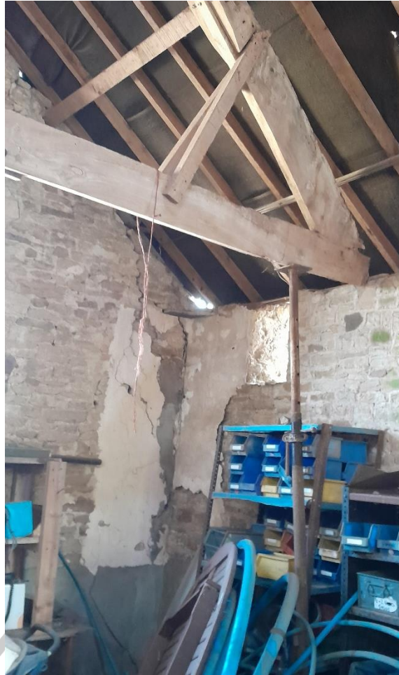
Photo 4: Propping of northwest truss
