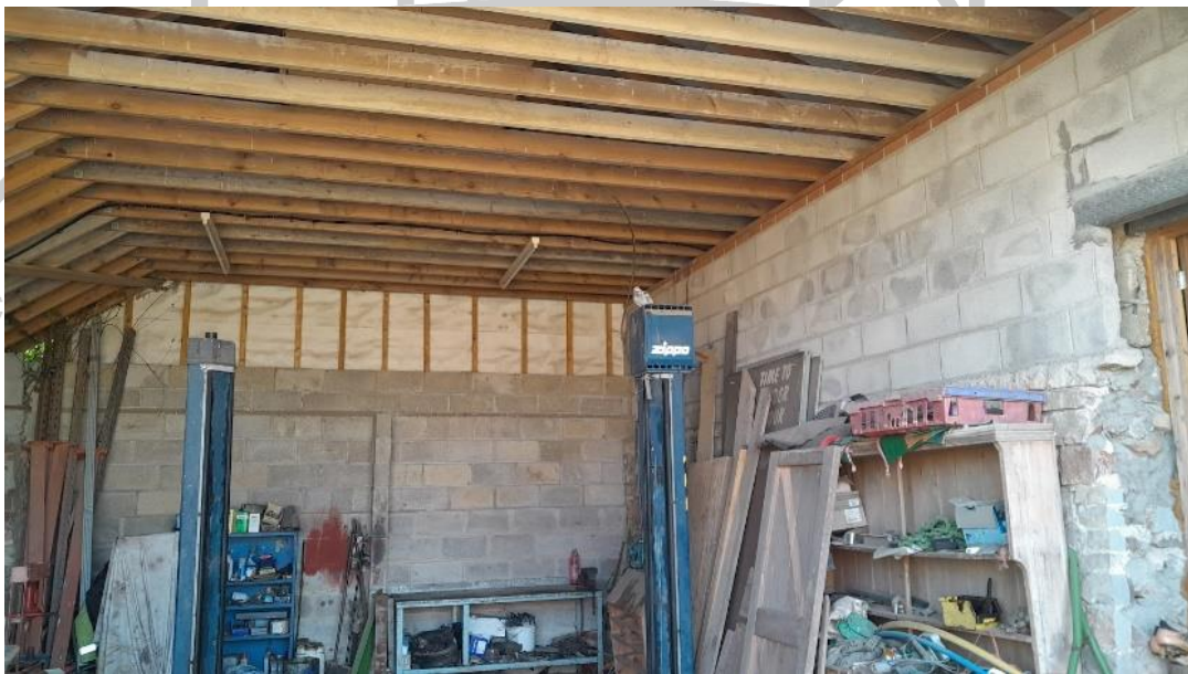
Photo 16: Internal view of blockwork wall and timber frame.
