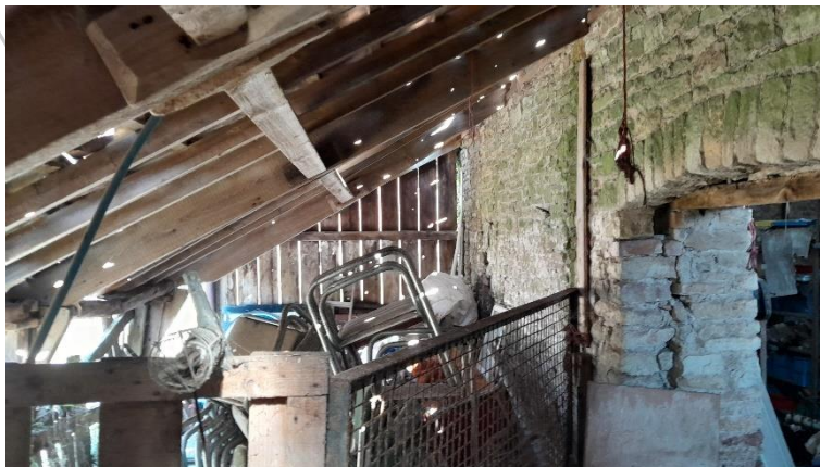
Photo 5: Southwest lean-to internal roof
