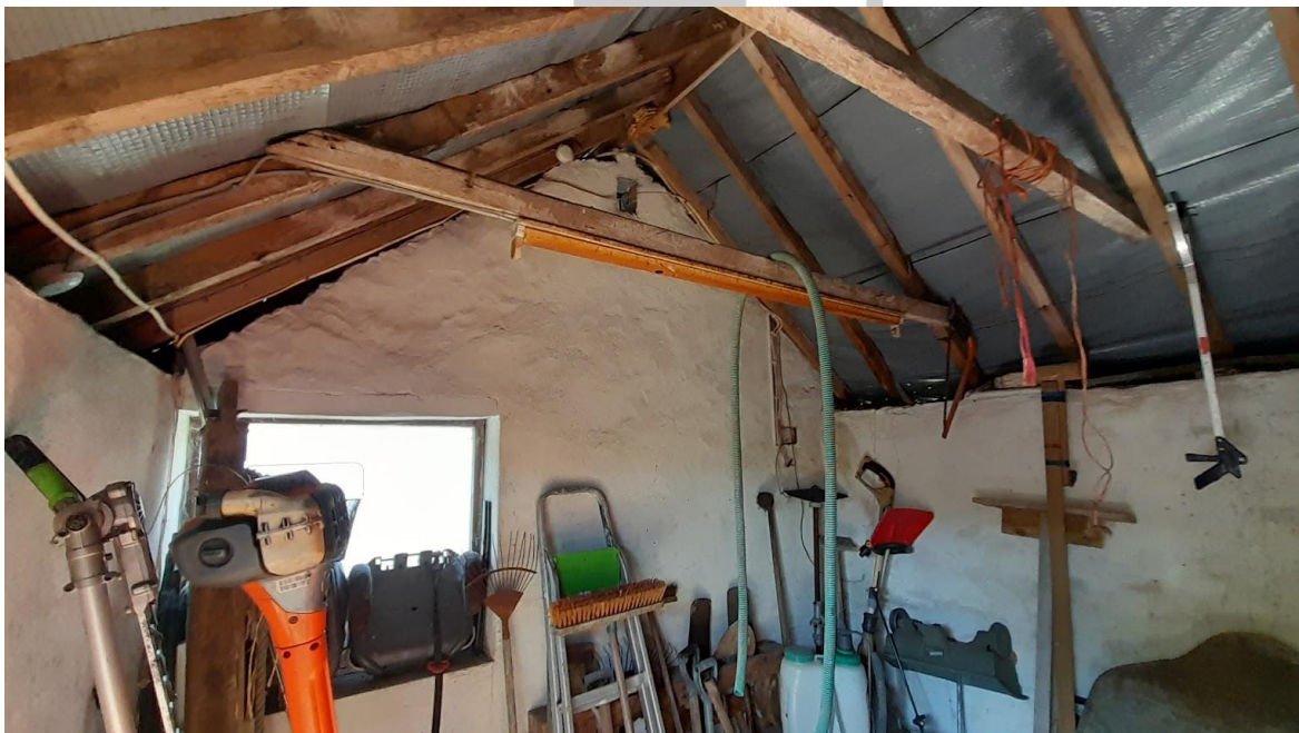
Photo 22: Internal view of barn
