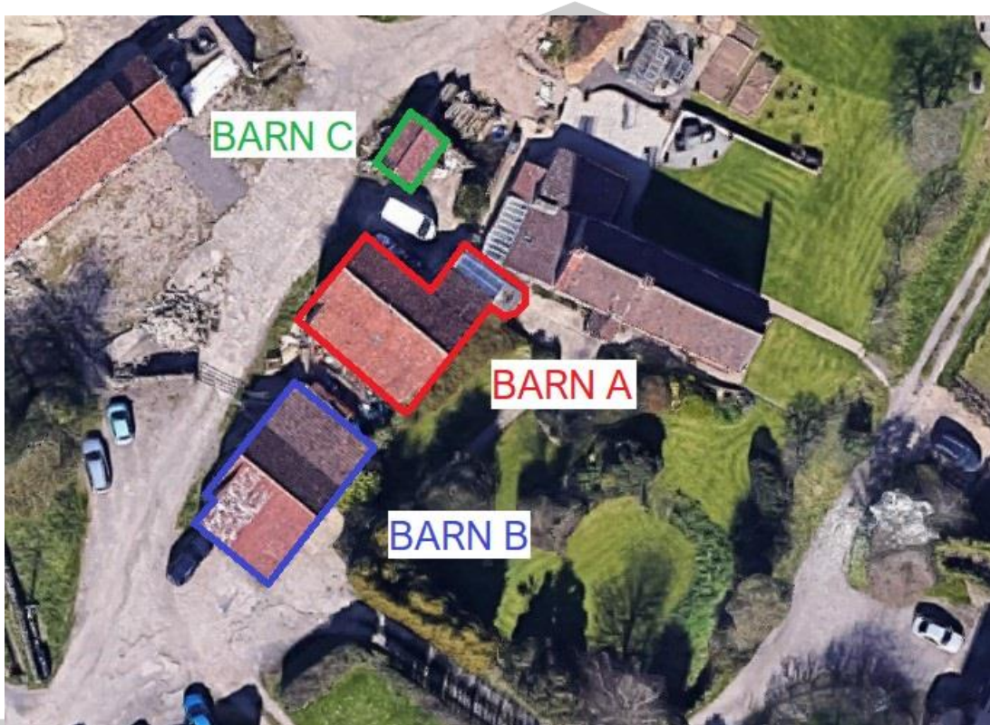
Figure 1: Aerial photograph of the barns
