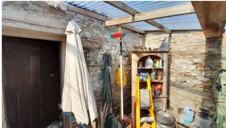
Photo 6: Northeast lean-to internal roof
