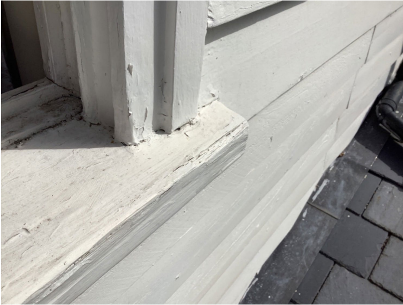
Figure 10 Window W4 Cill closeup
