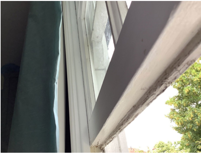
Figure 6 Window W2 Sash
