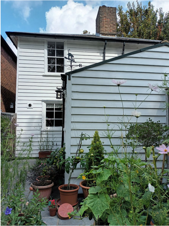
Figure 2 Rear Elevation, W3 and W4
