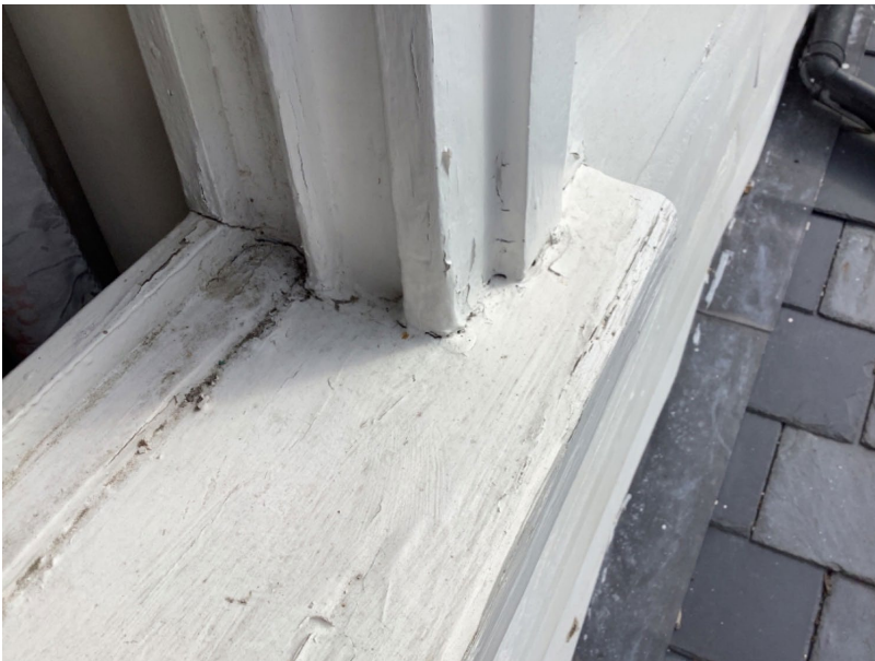
Figure 9 Window W4 Cill
