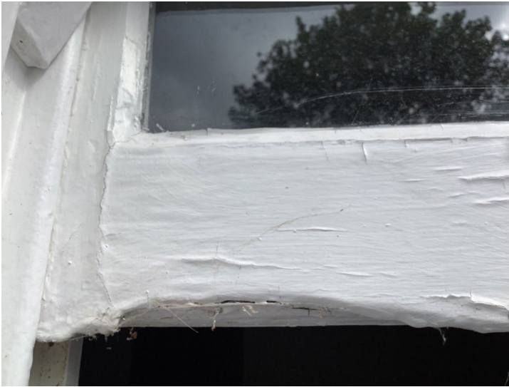
Figure 11 Window W4 Sash
