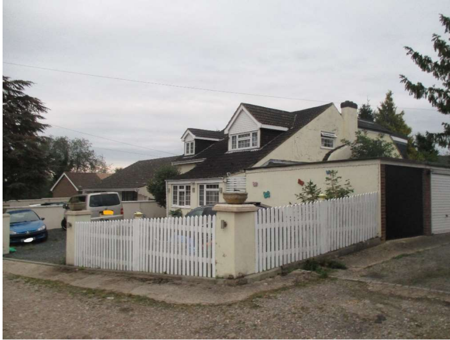
Neighbours property with well designed dormers
