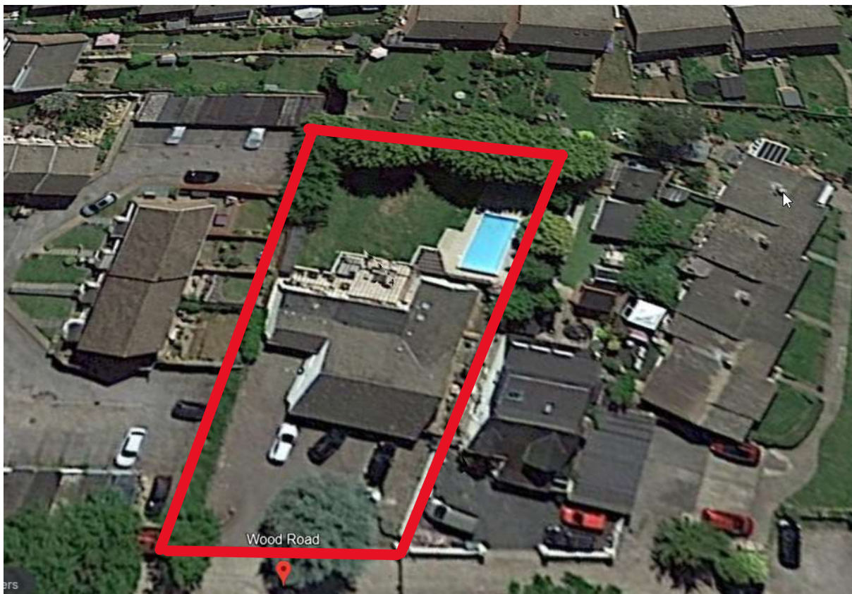
Aerial View of The Birches
