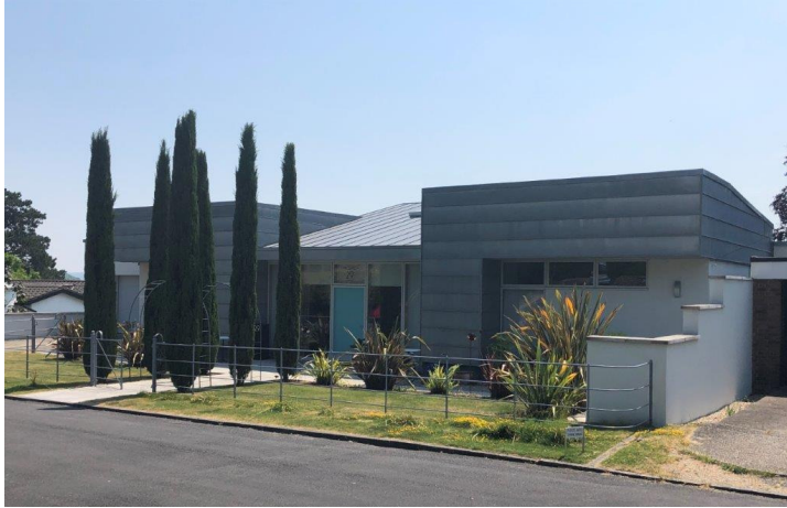
A substantial contemporary style house at the western end of Guildown Avenue on the south side
