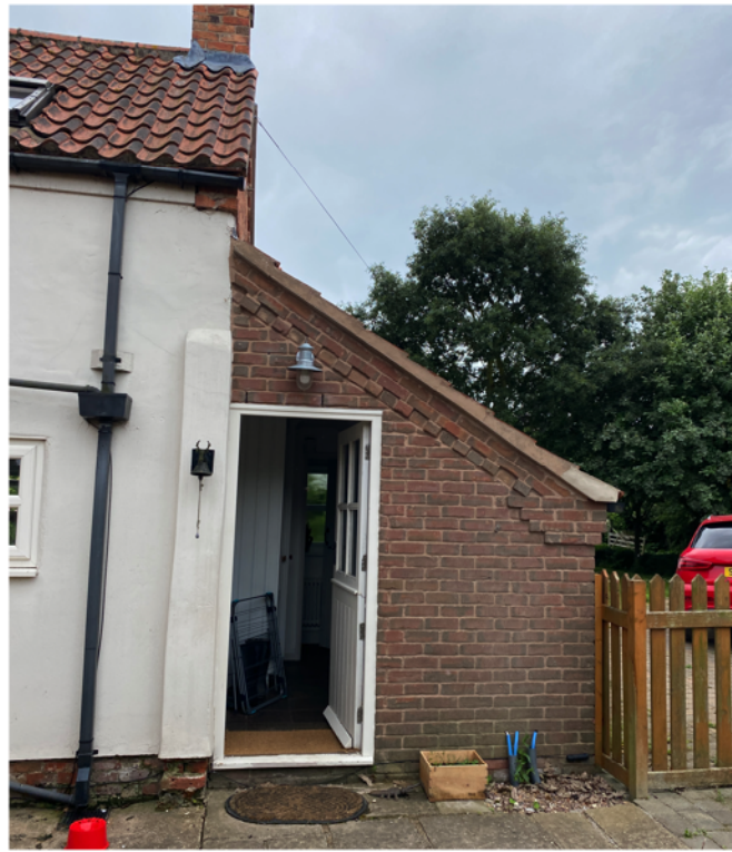
View of rear entrance from North West garden.
