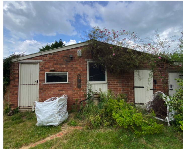
View of outbuilding in garden.
