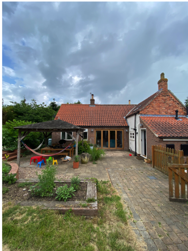
View of garden and North West elevation.
