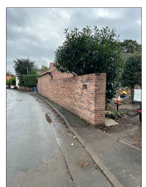
AS-BUILT WEST WALL NORTH EAST VIEW
