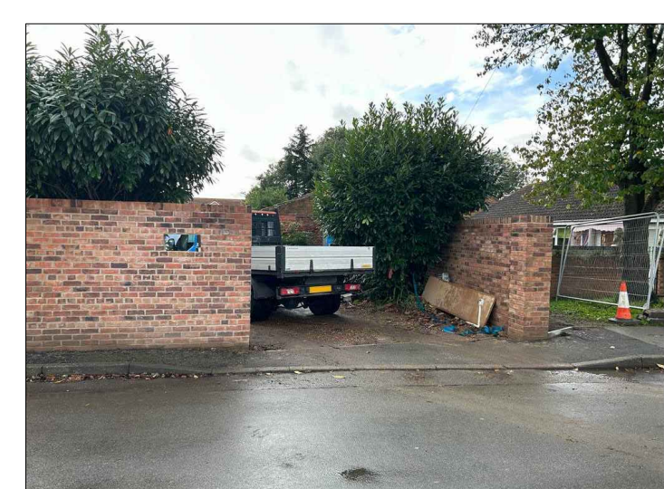
AS-BUILT WEST WALL EAST VIEW
