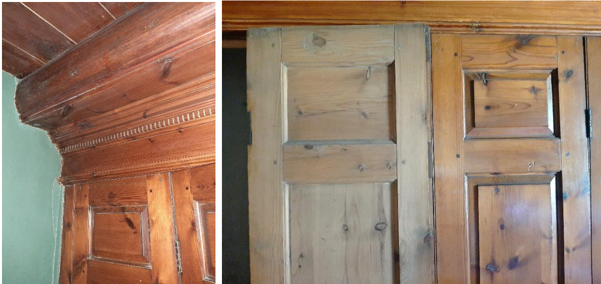
Joinery details : left - cornice, etc.; right – panels
