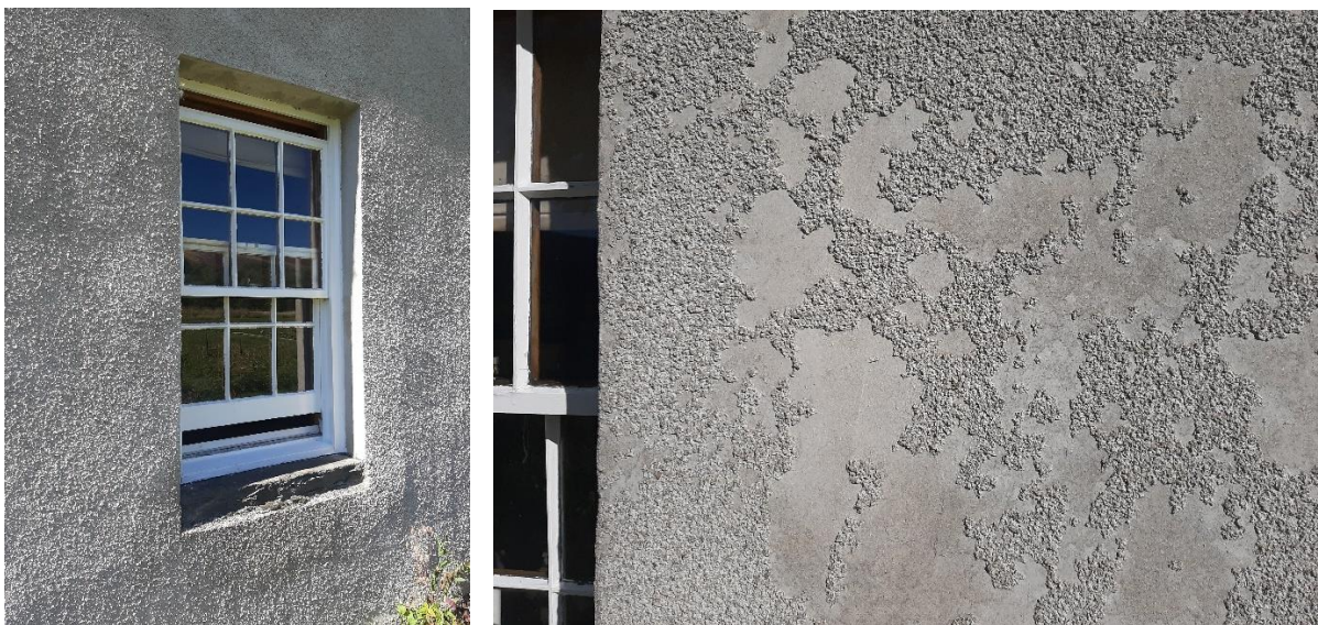
East elevation – detail of harl application at ground floor window
