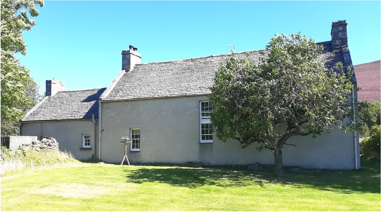
View of the rear (west) side of Ballantruan farmhouse
