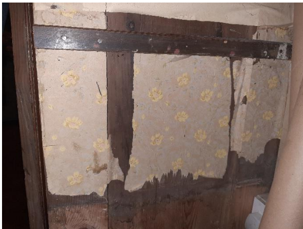
Left - wall-papered interior of western box bed, paper onto timber lining boards terminating at top of bed-frame below, now missing; right – paper lining visible within eastern box bed
