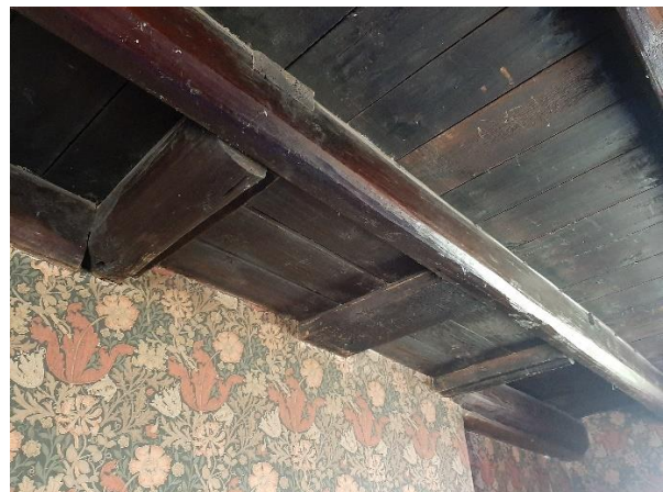
Detail of ceiling structure – light dressing of joists with a draw-knife; right – framing for the first floor fireplace hearth-stone to the north wall
