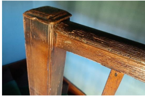
Detail of balustrade – newel, rail and baluster
