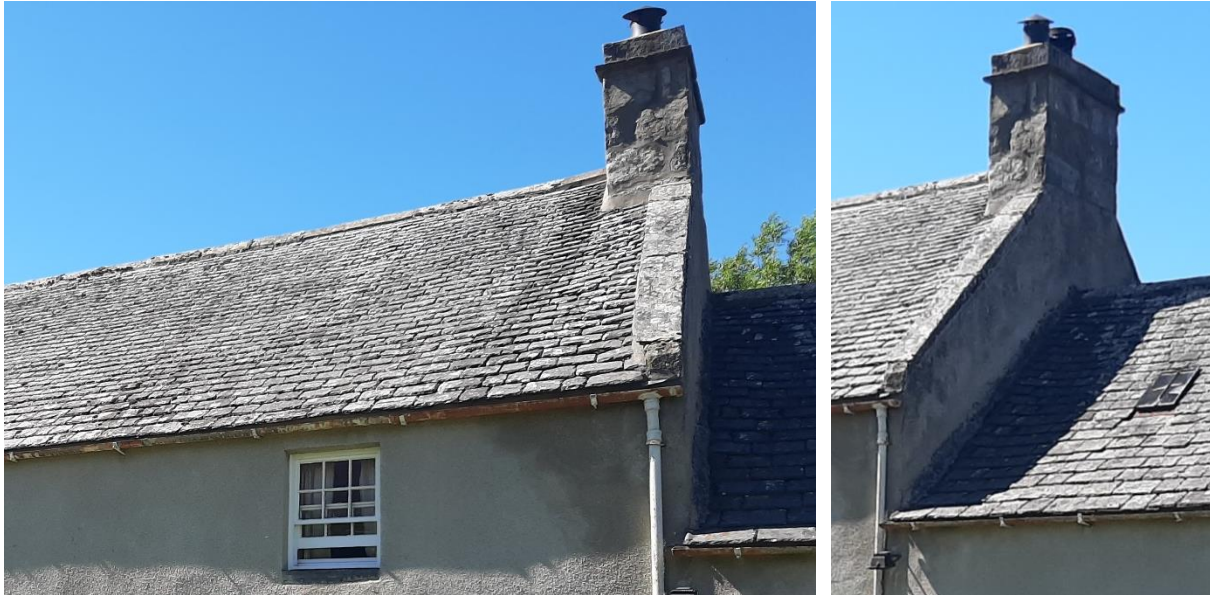
Main house – roof details, slating, gable head and chimney
