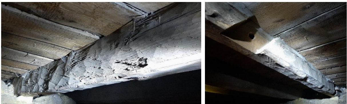
Detail showing adze-dressing to roof timbers
