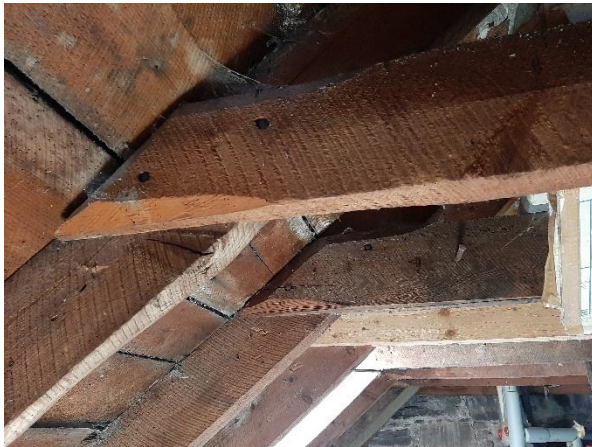
Left – detail of collar joint; right – detail of apex jointing
