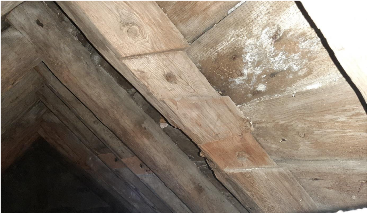
Detail showing relict collar joints – the upper with some weathering, the lower more recently exposed, both pegged
