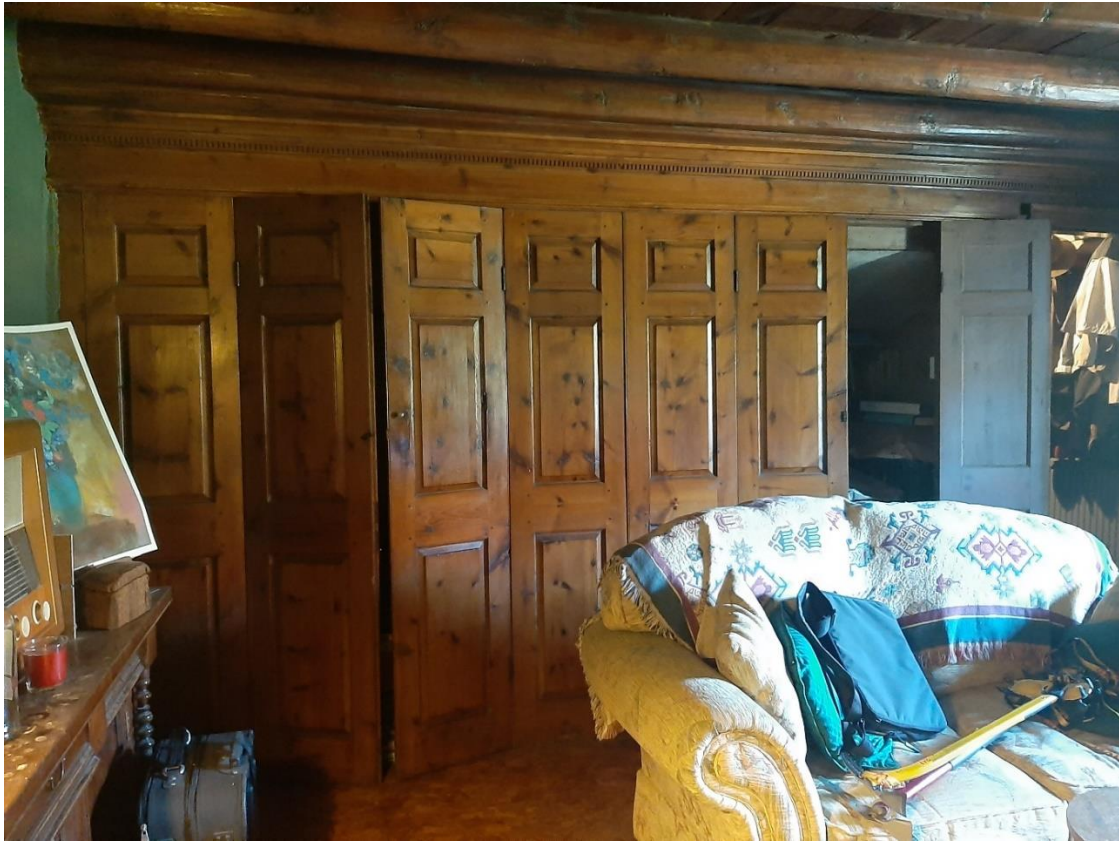
North wall showing arrangement of panelling incorporating paired doors to two box beds
