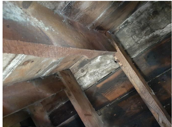
Left – detail of collar joint; right – detail of apex jointing
