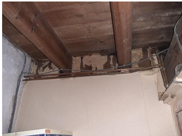
Left - wall-papered interior of western box bed, paper onto timber lining boards terminating at top of bed-frame below, now missing; right – paper lining visible within eastern box bed
