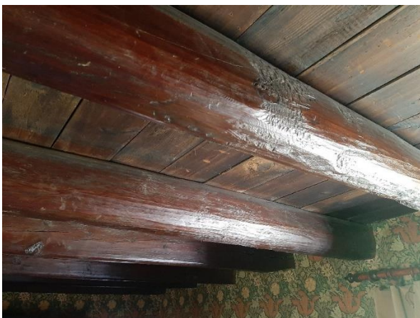
Detail of ceiling structure – light dressing of joists with a draw-knife; right – framing for the first floor fireplace hearth-stone to the north wall
