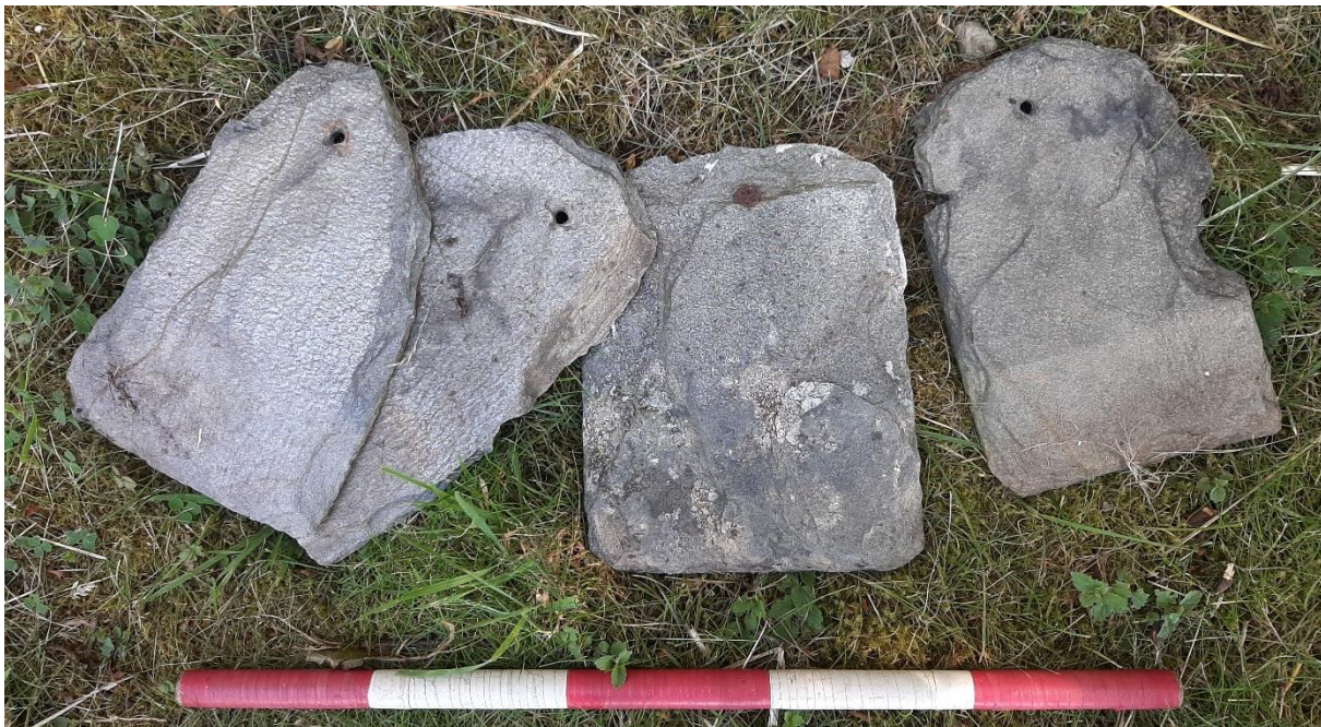
Ex situ 'Tomintoul' slates at site, some retaining wrought iron nails, some with mortar residues
