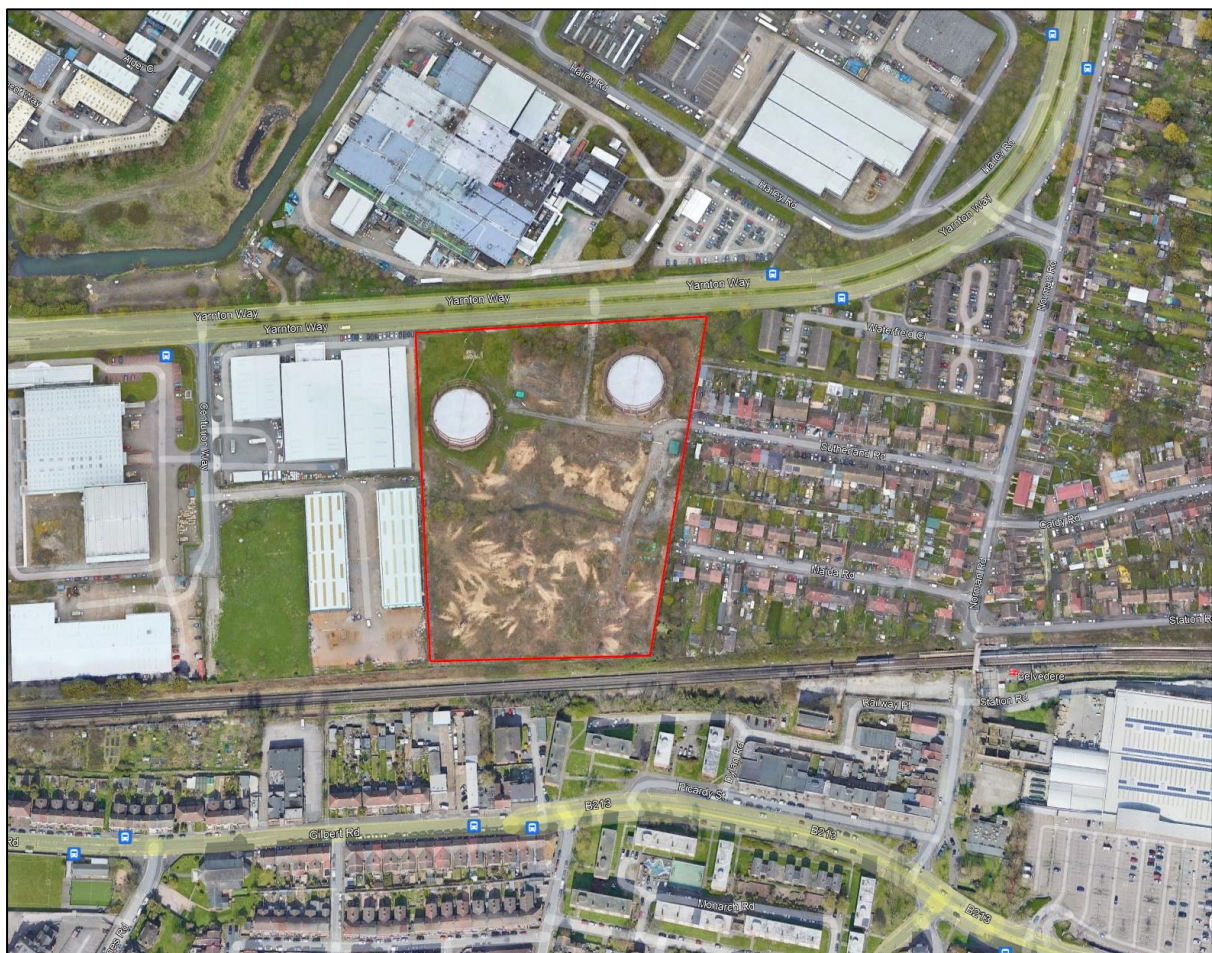
Figure 1-1: Site Boundary and Surrounding Area
