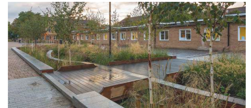
Exposed water course
