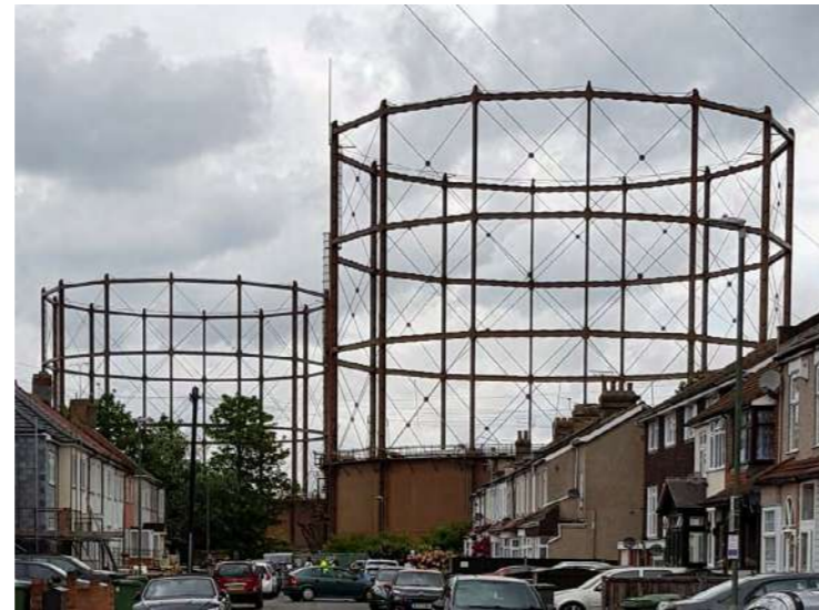
Image taken prior to dismantling of gas holders
