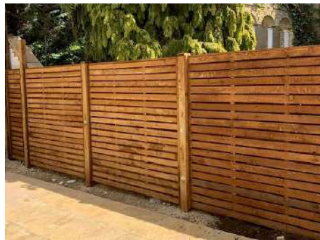
Timber fence to rear gardens
