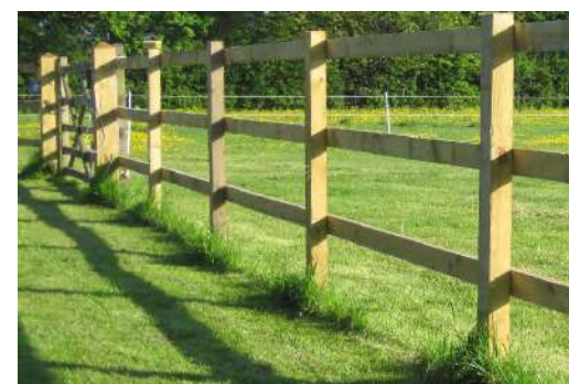
Timber post and rail fence to the area safeguarded for Tiny Forest initiatives
