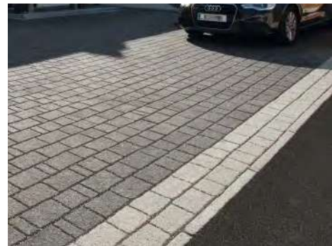
Permeable block paving
