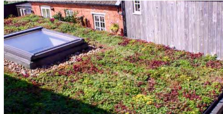
Extensive roof with sedum planting
