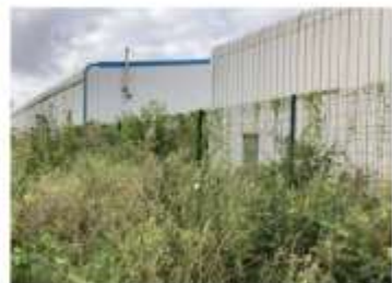
Adjacent warehouses through boundary fence
