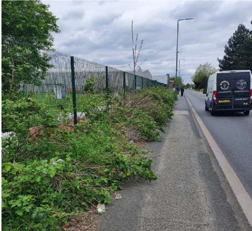
Key Journey No. 1 – Photo (Southern Side of Yarnton Way on Site Frontage)
