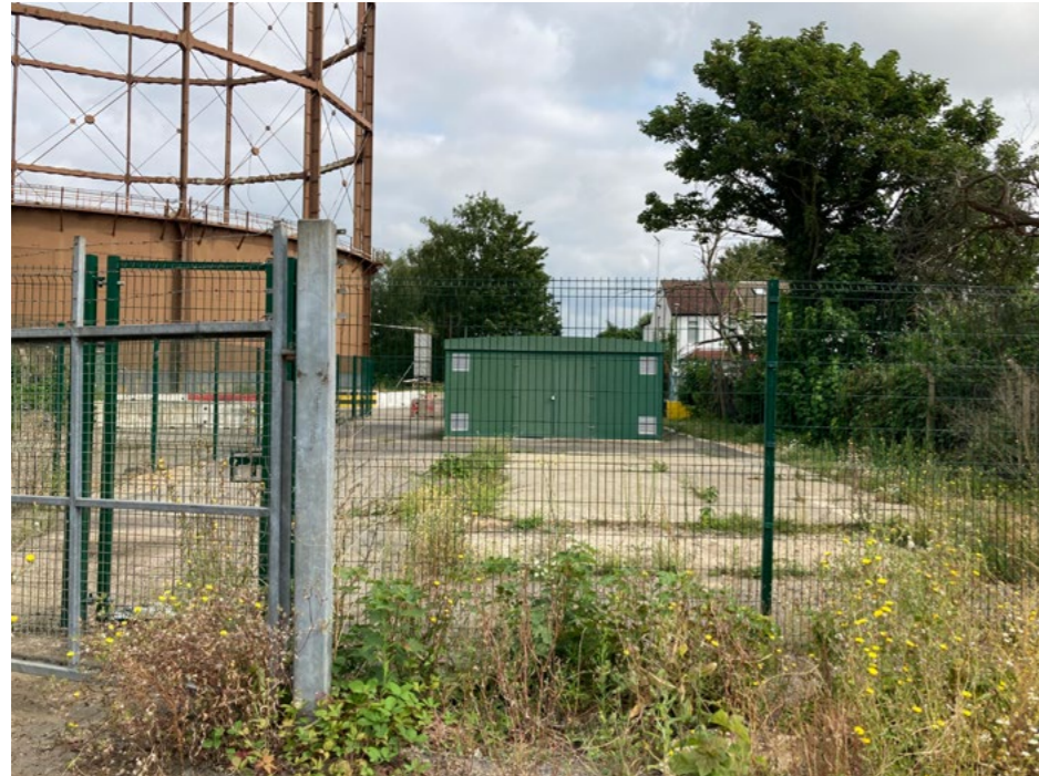
4. AREAS FOR GAS WORKING ARE CLEAR AND MAINTAINED
