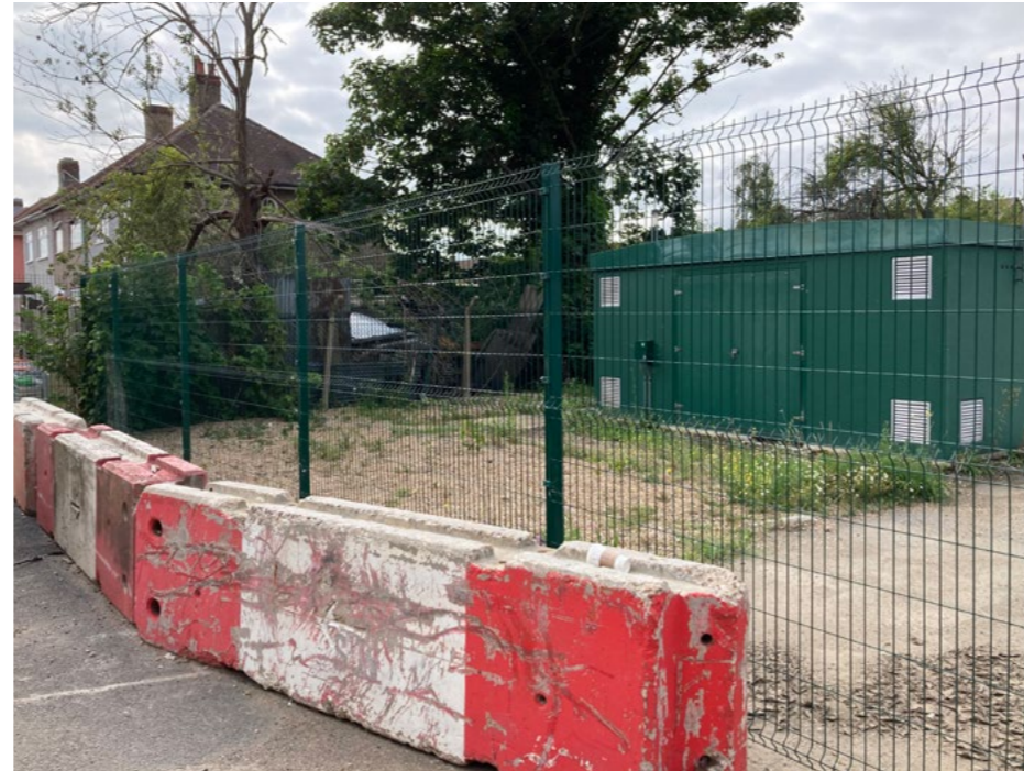
5. THE GAS GOVERNOR AND EASTERN ACCESS POINT FROM SUTHERLAND ROAD
