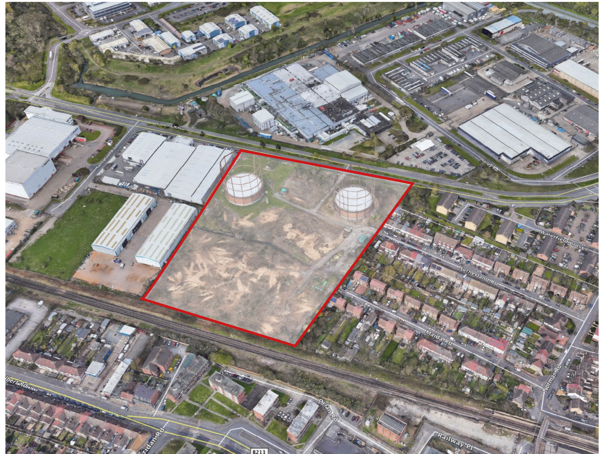
1. AERIAL VIEW OF THE SITE FROM THE SOUTH-EAST - NOTE: THE GAS-HOLDER ON THE RIGHT OF THE IMAGE HAS SUBSEQUENTLY BEEN DEMOLISHED
