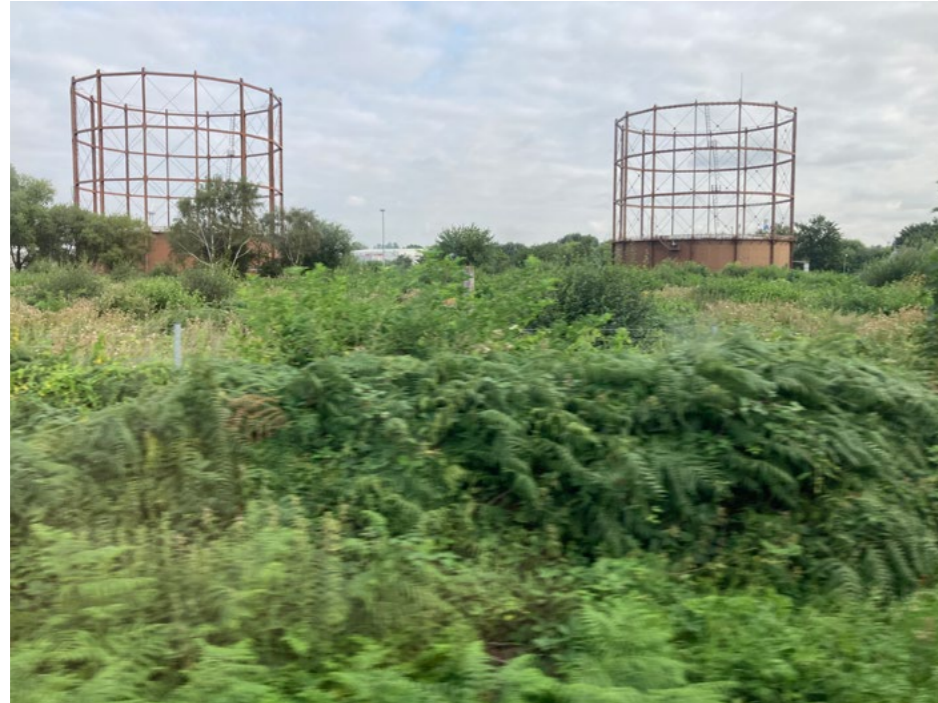
1. THE TWO GAS-HOLDERS SEEN THROUGH DENSE UNDERGROWTH
