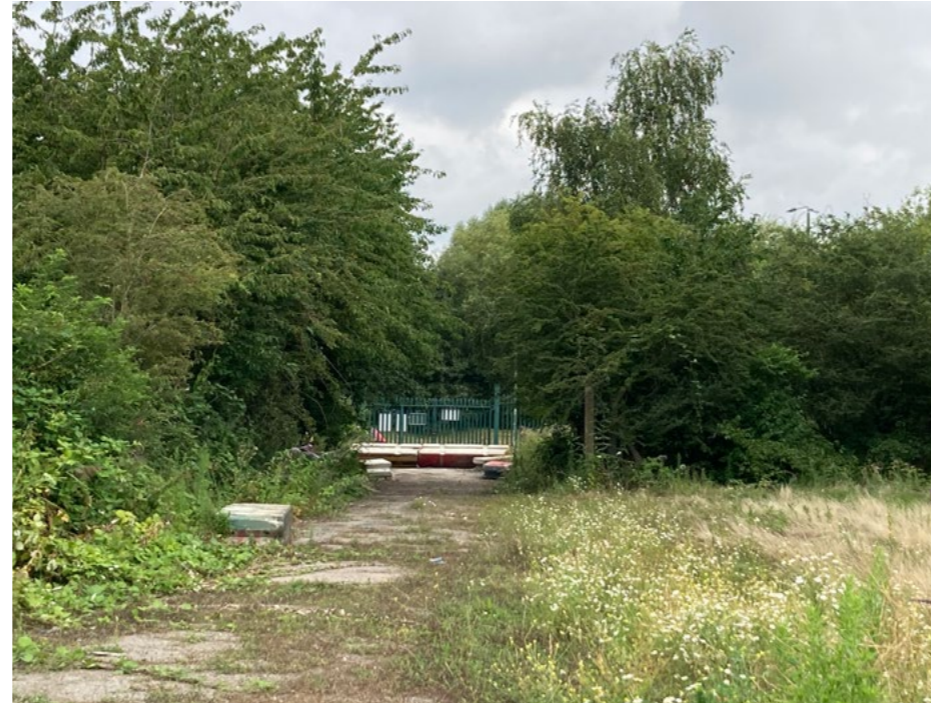
2. THE EXISTING ENTRANCE ON YARNTON WAY
