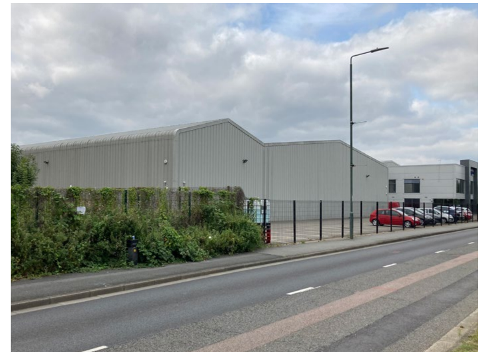
6. WAREHOUSES CENTRED AROUND CENTURION WAY
