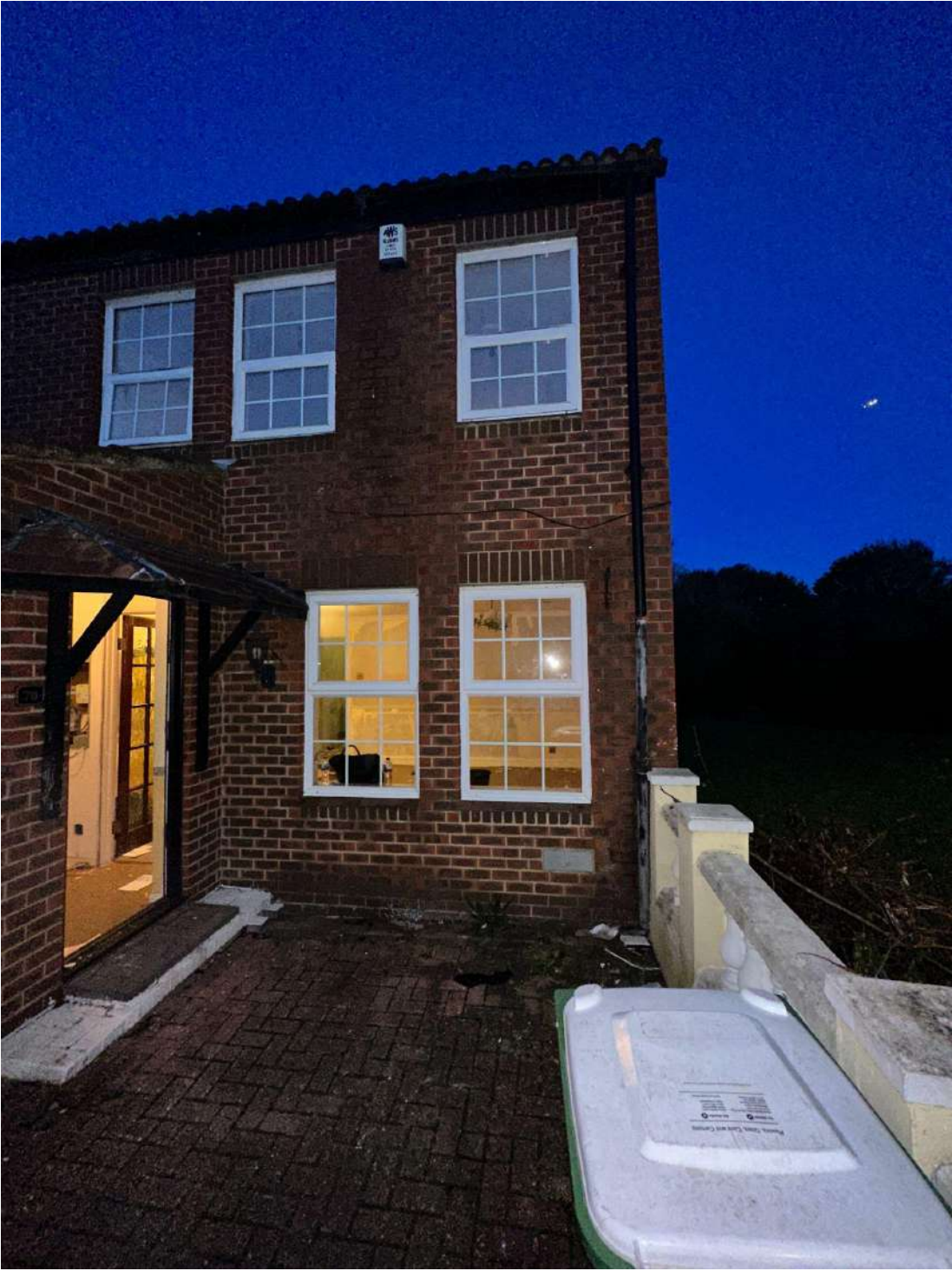
Image 04 - Front View of 70 Fieldfare Road, Bexley
