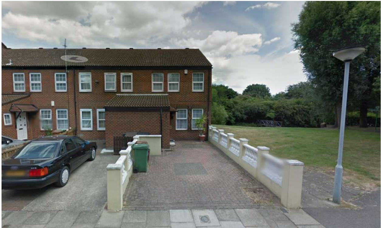
Image 01 - Front View of 70 Fieldfare Road, Bexley
