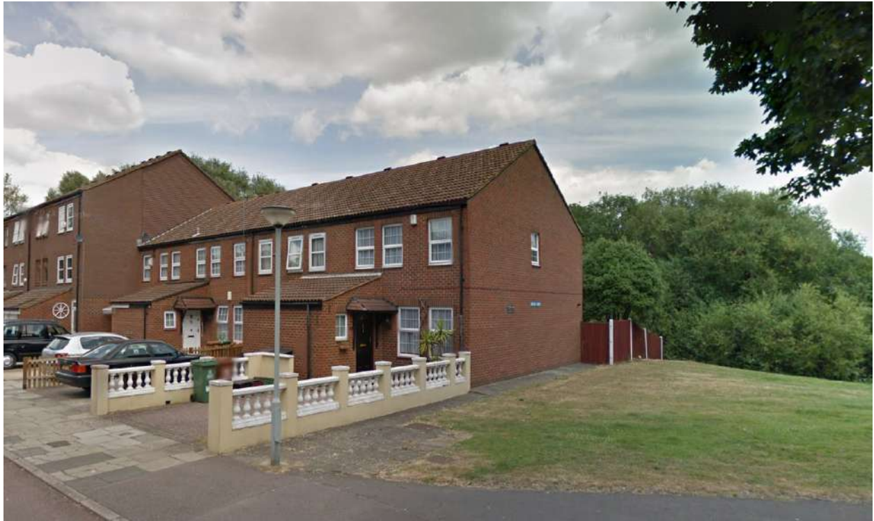
Image 02 - Front View of 70 Fieldfare Road, Bexley
