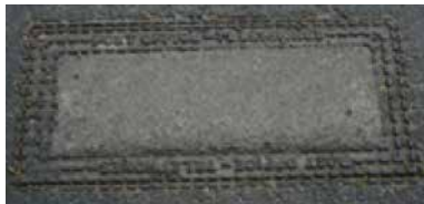
Old style cast iron and concrete 38x80cm
