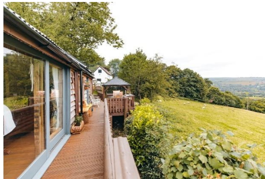
Figure 6 – Image of lodge exterior.
