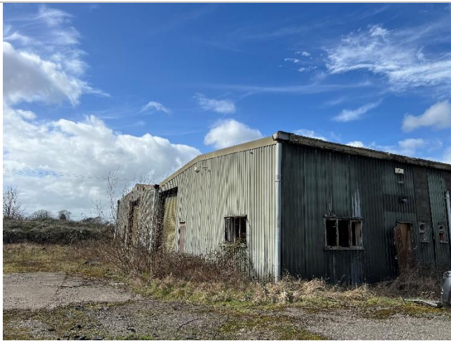
View of the building near the south-east corner of the site.
