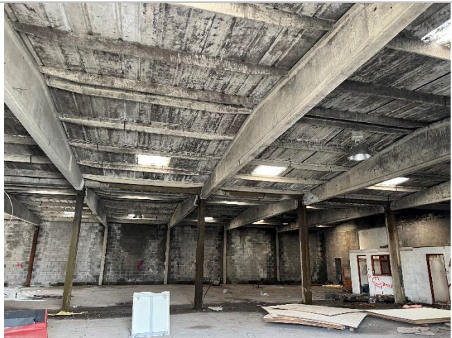
Internal view of the building with precast concrete support beams.
