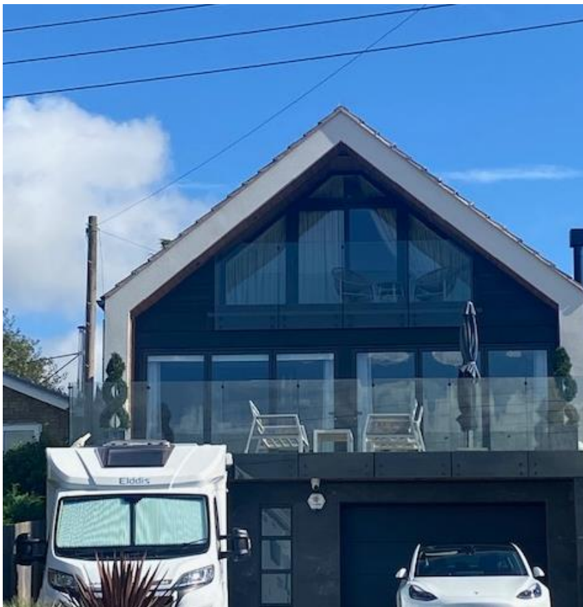
Glazed gable and balcony – 393 Nore Road
