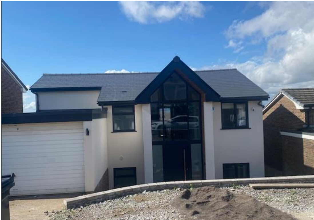
Glazed gable – 82 Hillside Road
