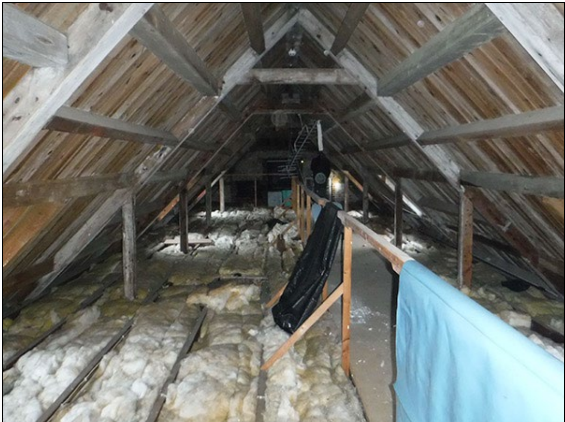
Figure 24 The roof of the mill, looking north-east
