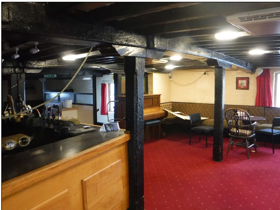
Figure 11 View of the first floor showing the two cambered and moulded transverse beams at its north-eastern end, probably re-used ships timbers
