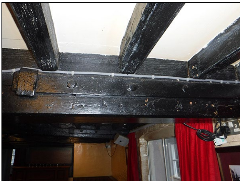
Figure 29 One of the metal straps attached to the transverse beams
