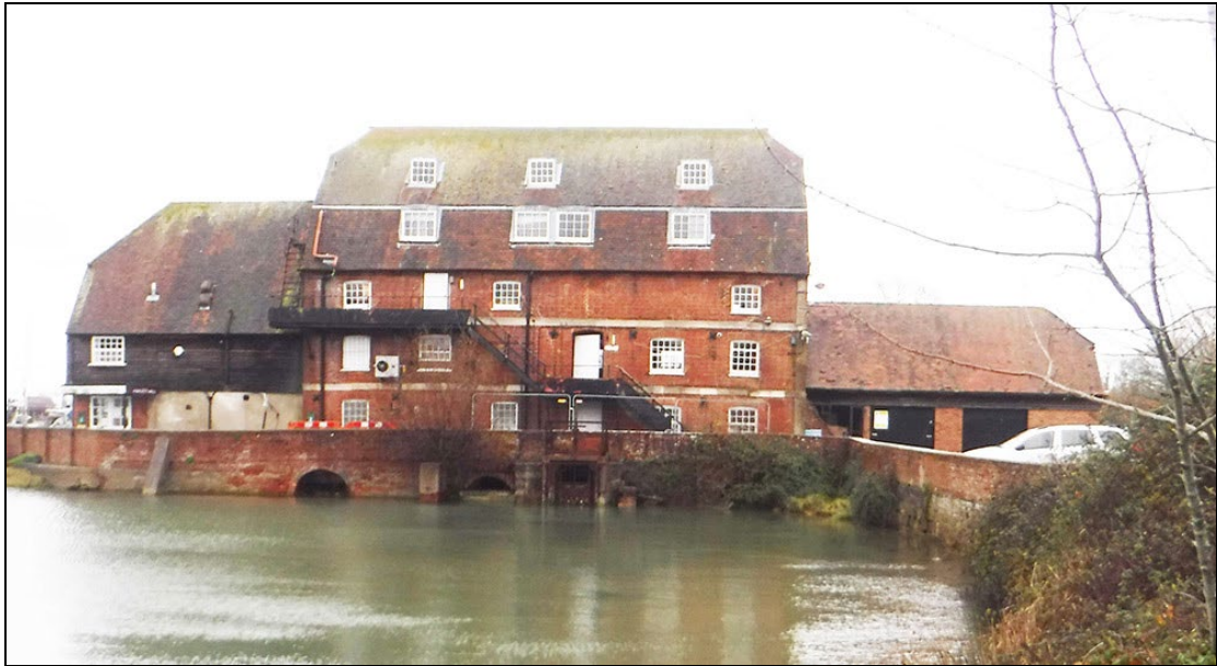
Figure 8 The northwest elevation of Ashlett Mill
