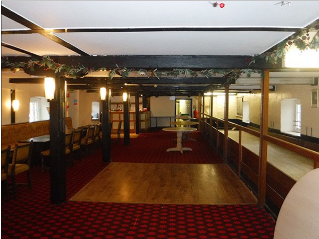
Figure 10 View of the second floor looking north-east, showing the transverse beams supported on their posts, although the right hand posts are all replacements linked to the skittle alley (and probably shooting range before)
