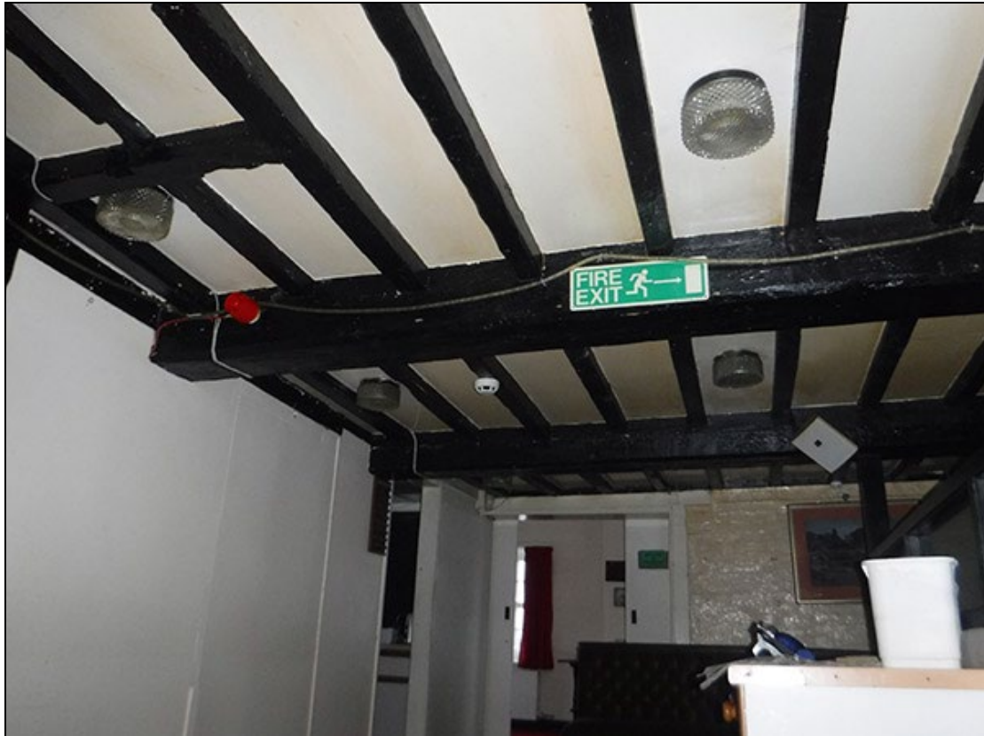
Figure 14 Two of the transverse beams in the northern extension, looking northeast
