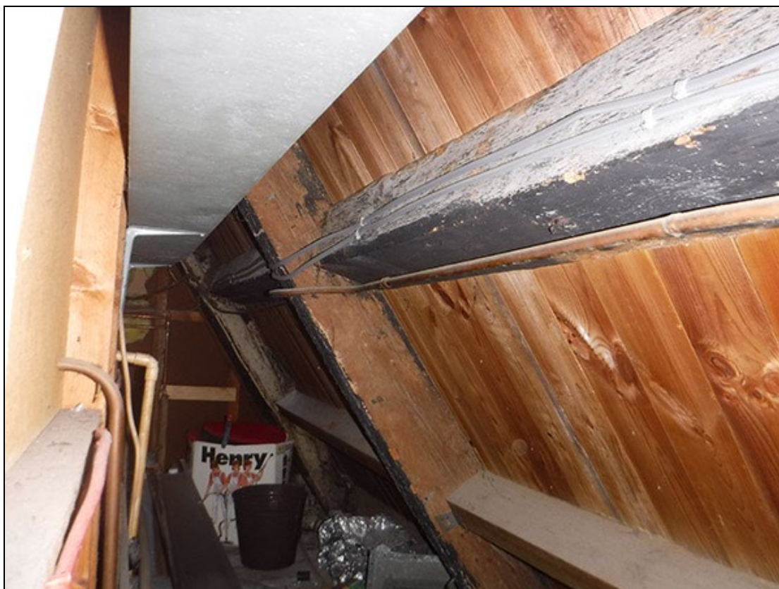
Figure 18 The roof of the northern extension, looking southwest
