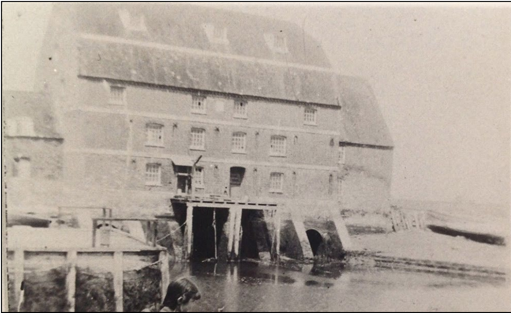
Figure 25 The southeast elevation of Ashlett Mill c.1910 (HRO No.70A09/4/48/1)
