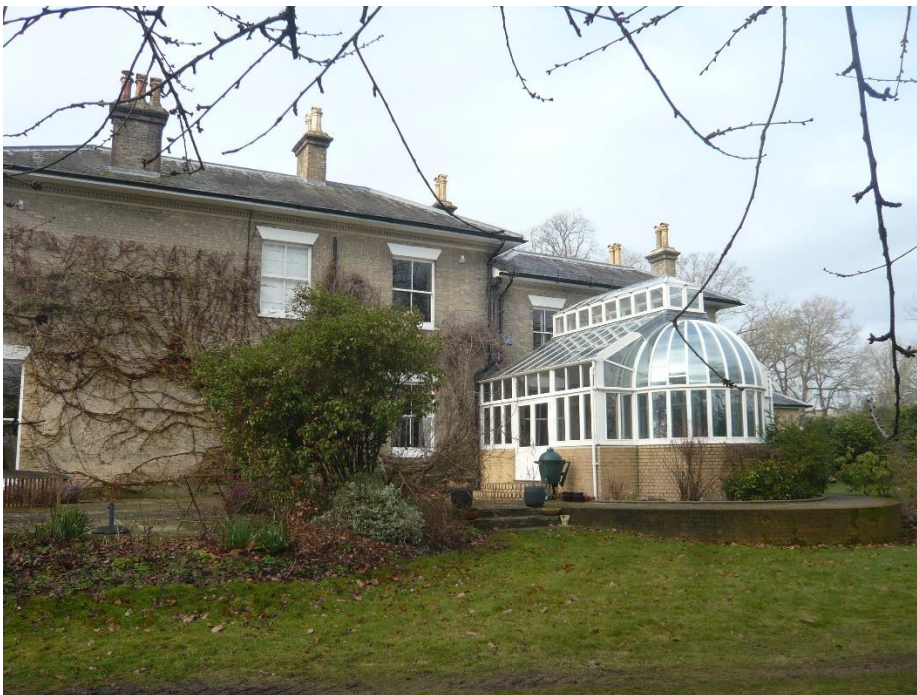
Fig.6 Conservatory on the east side of the house
