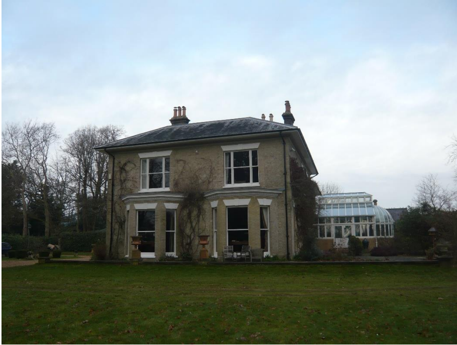
Fig.5 South side of the house
