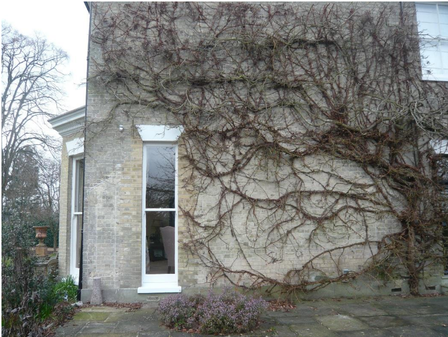
Fig.8 Window in position of a former door and scarring in the brickwork on the east side of the house where a previous structure stood
