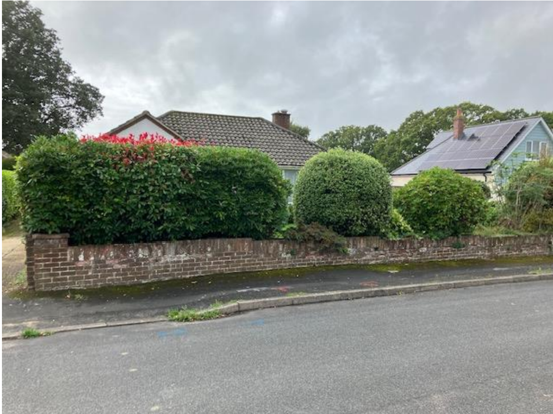
Front boundary wall showing dropped kerb wider than existing driveway.
