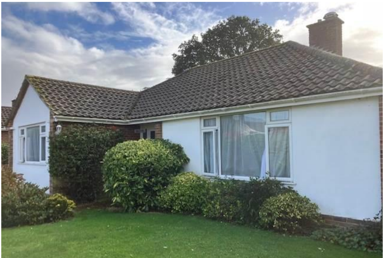
Fig 4 Front of house showing position for Porch to front door set back from forward Gable
