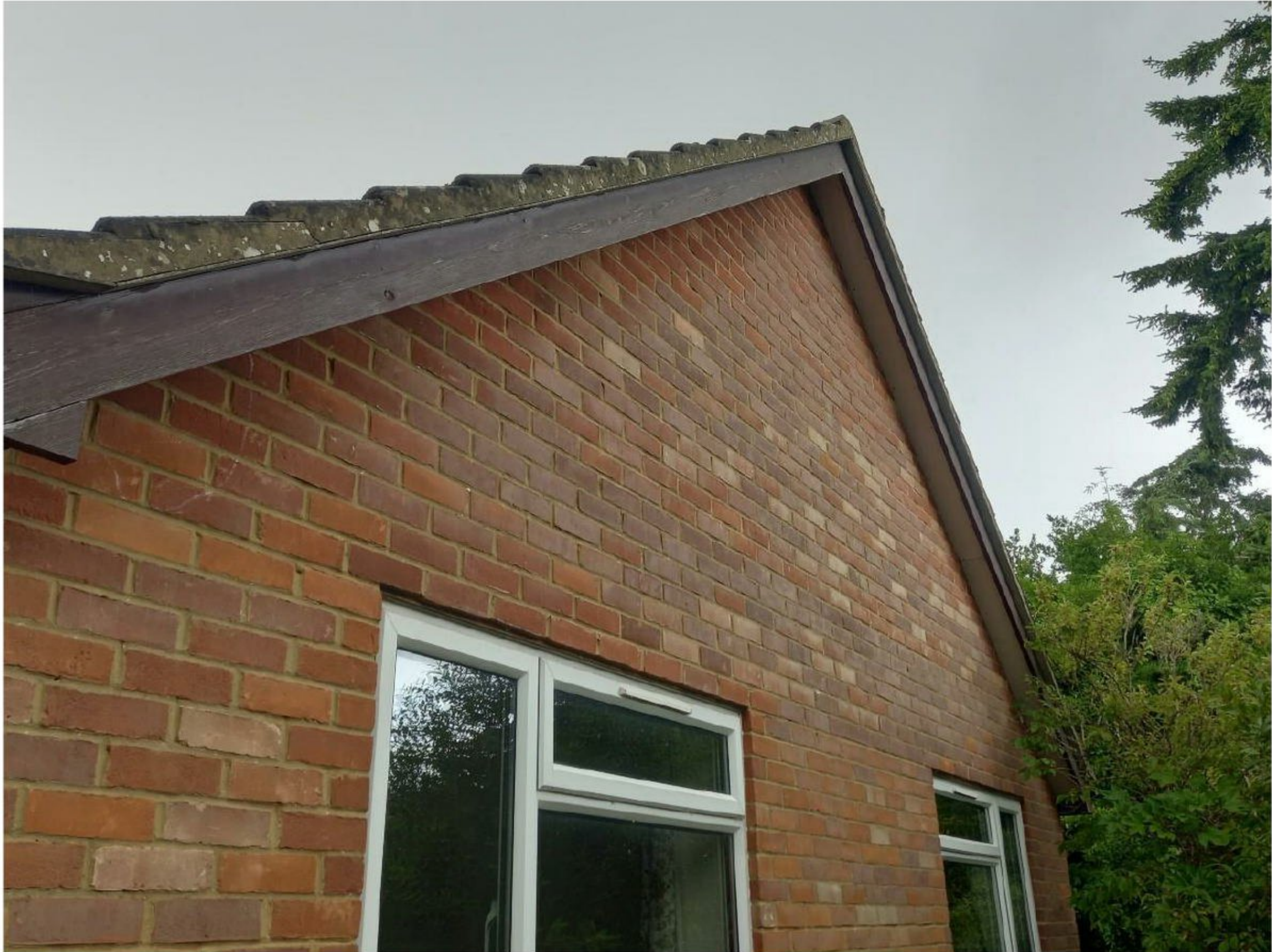
Plate 7 – Northern aspect of building 1.
