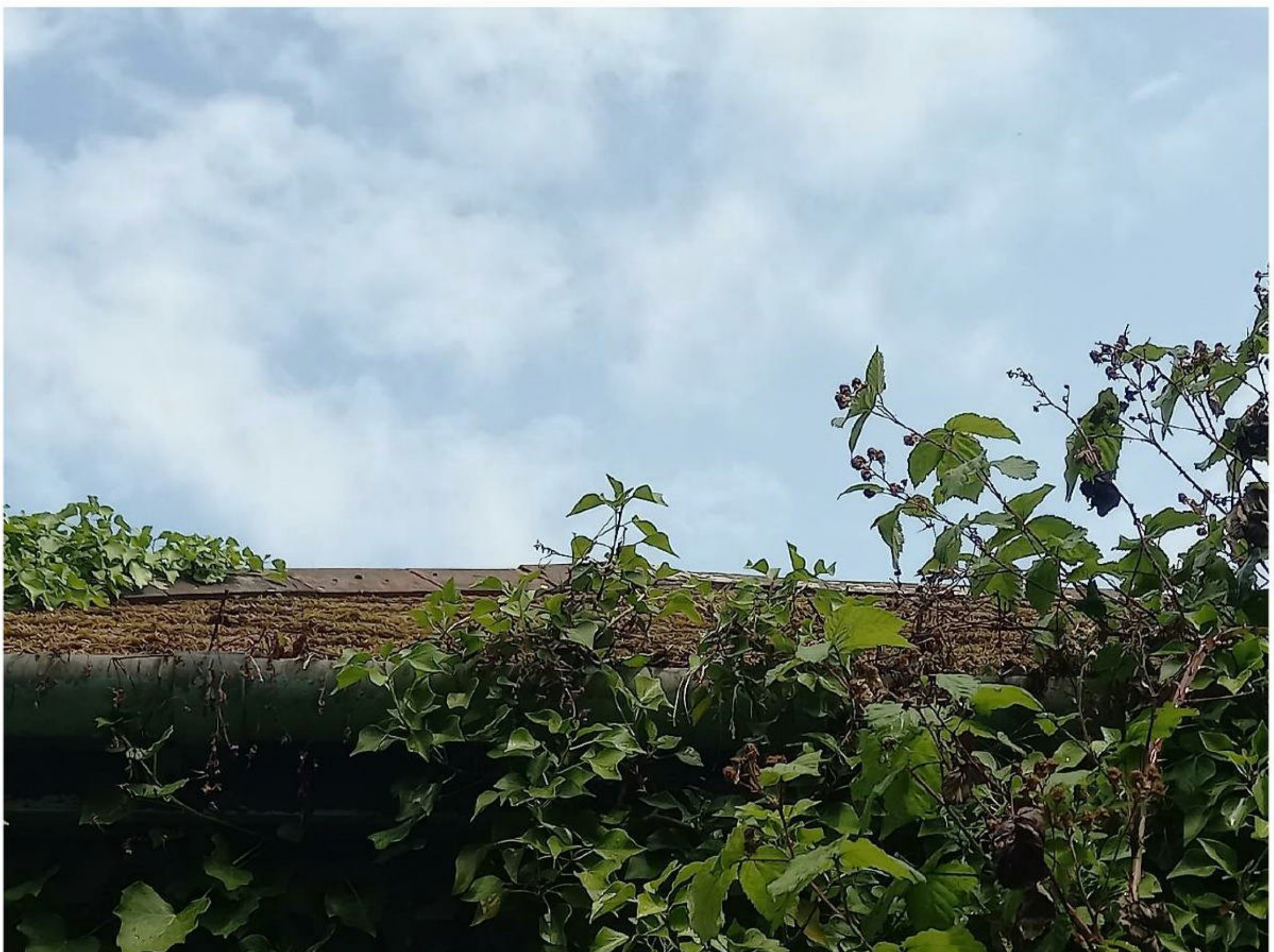
Plate 16 – Roof of building 4.
