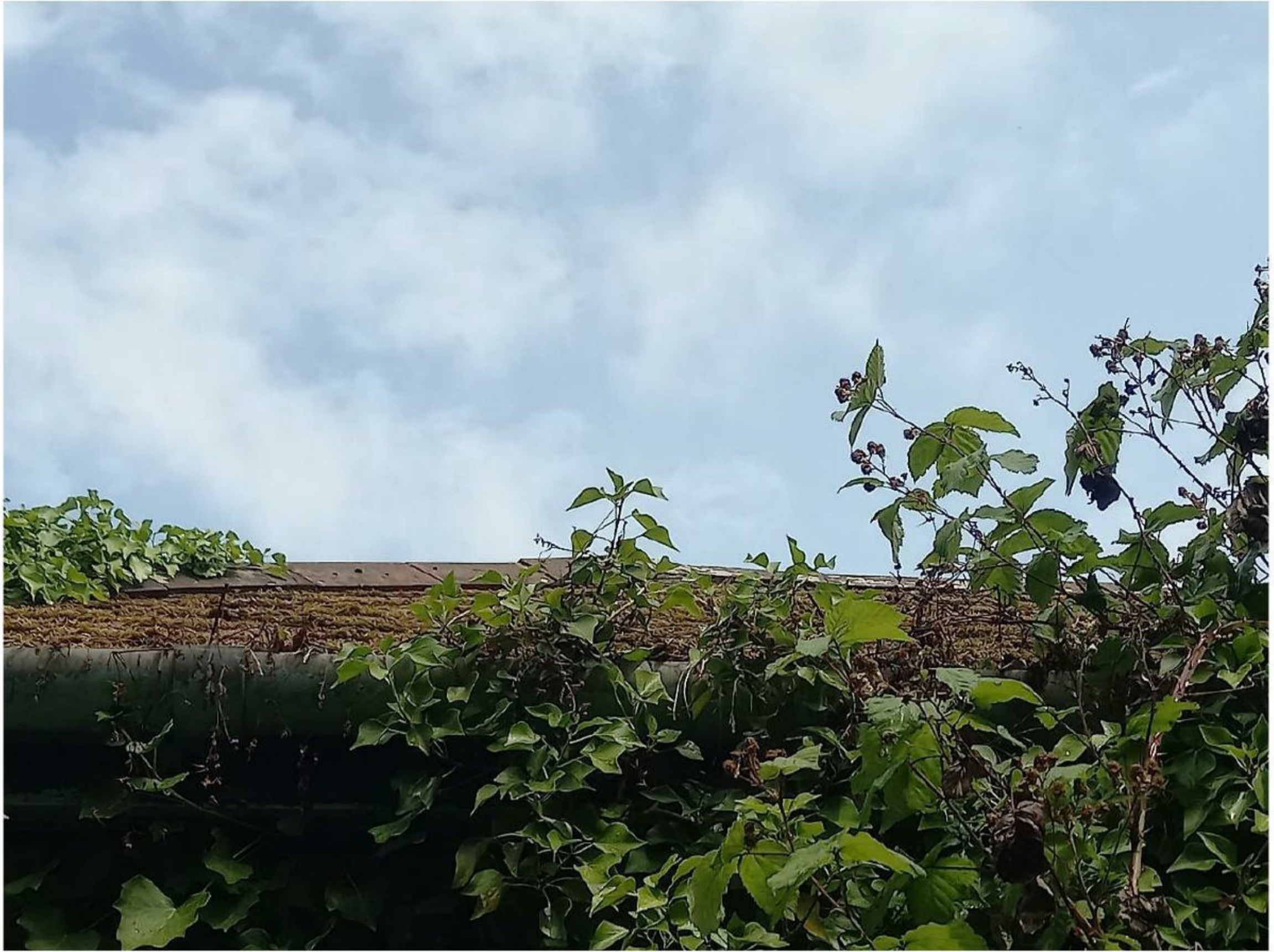
Plate 15 – Roof of building 4.
