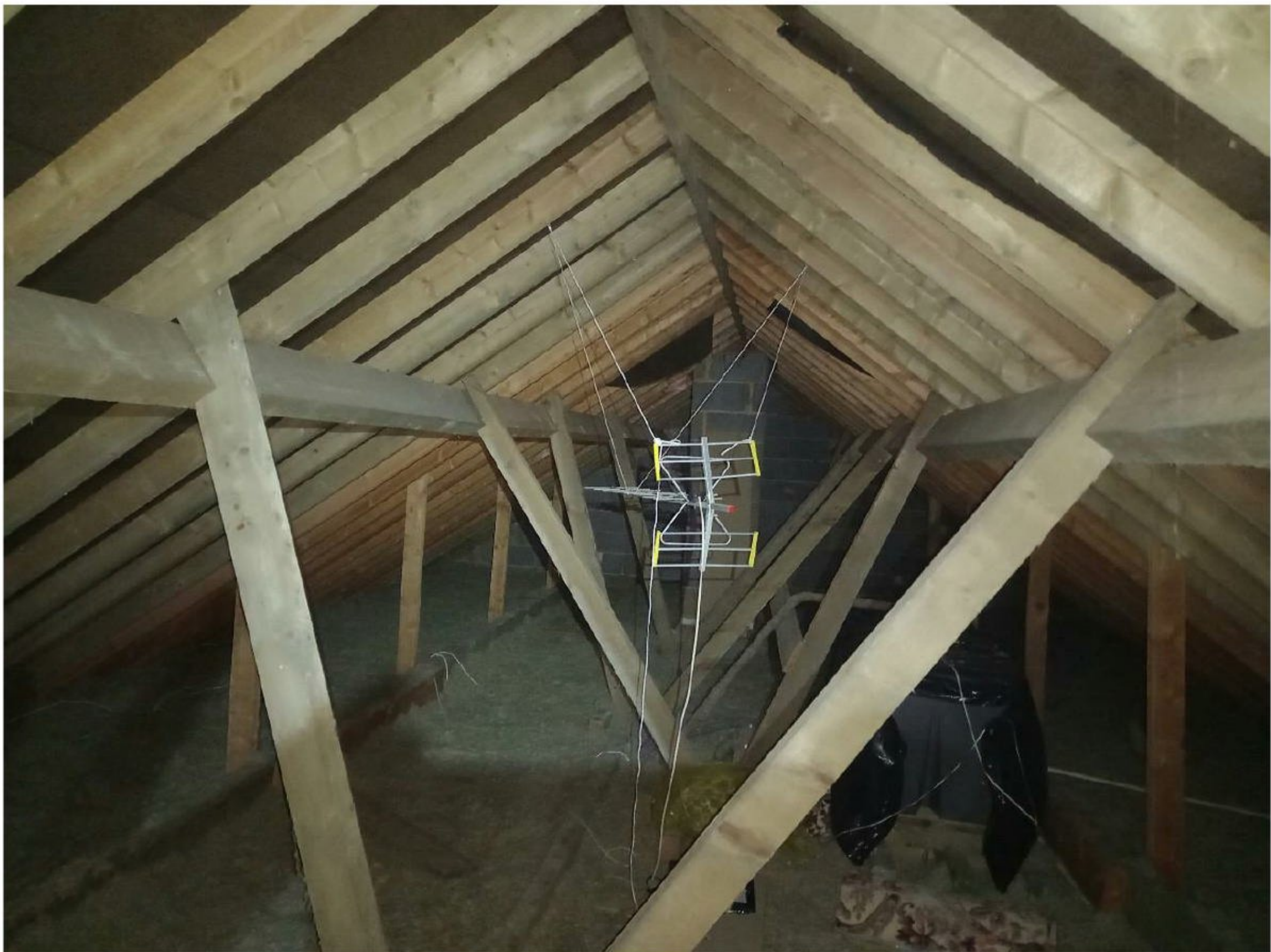
Plate 2 – Internal Photograph of the loft space in building 1.
