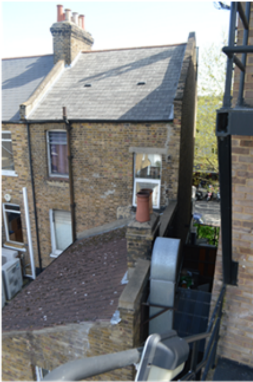
Rear Elevation of 54 Lordship Lane
