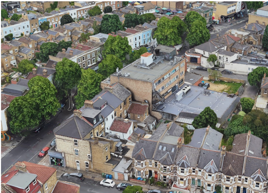
Aerial View from the North showing the large dominant flank wall to 56-60 Lordship Lane.
