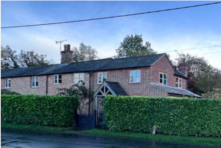
View of the front of Number 7 Sheldon Road
