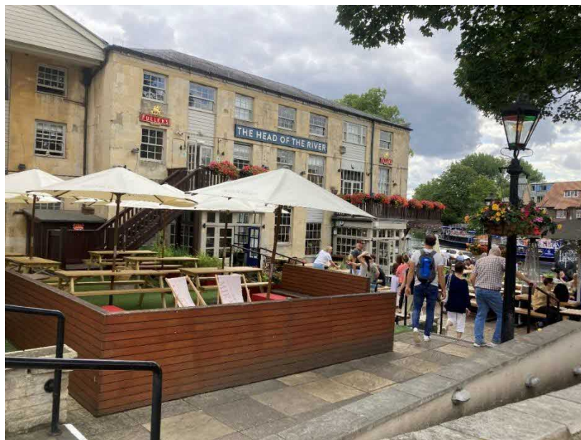
Above – Existing front wall of former warehouse and existing timber boxed enclosure within recess of front wall behind staircase
