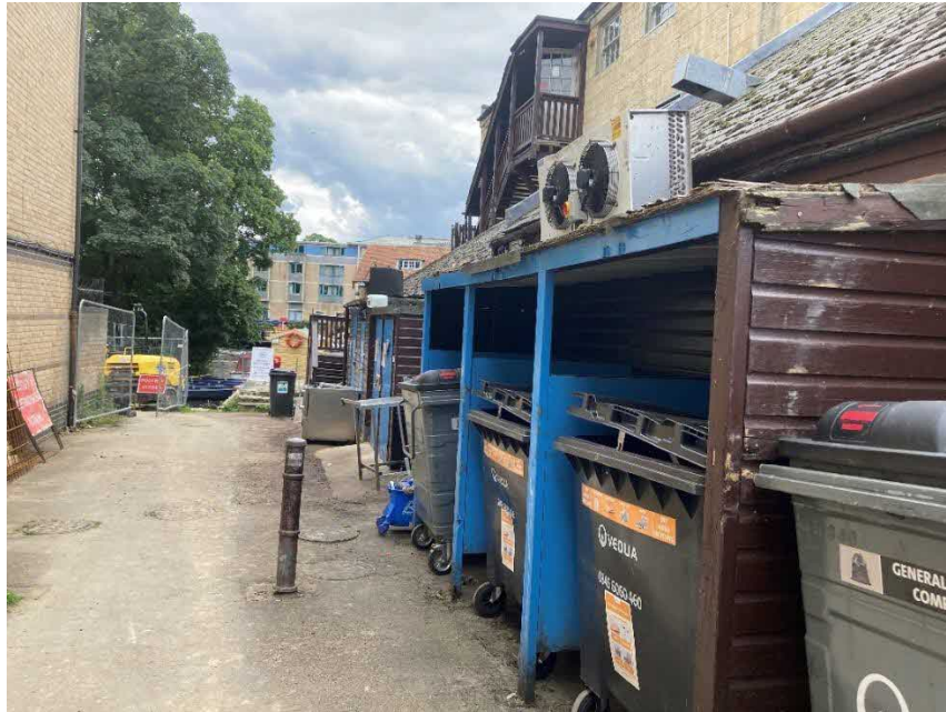
Above – Existing open bin store enclosures
