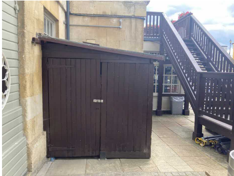
Above – Existing timber enclosure
