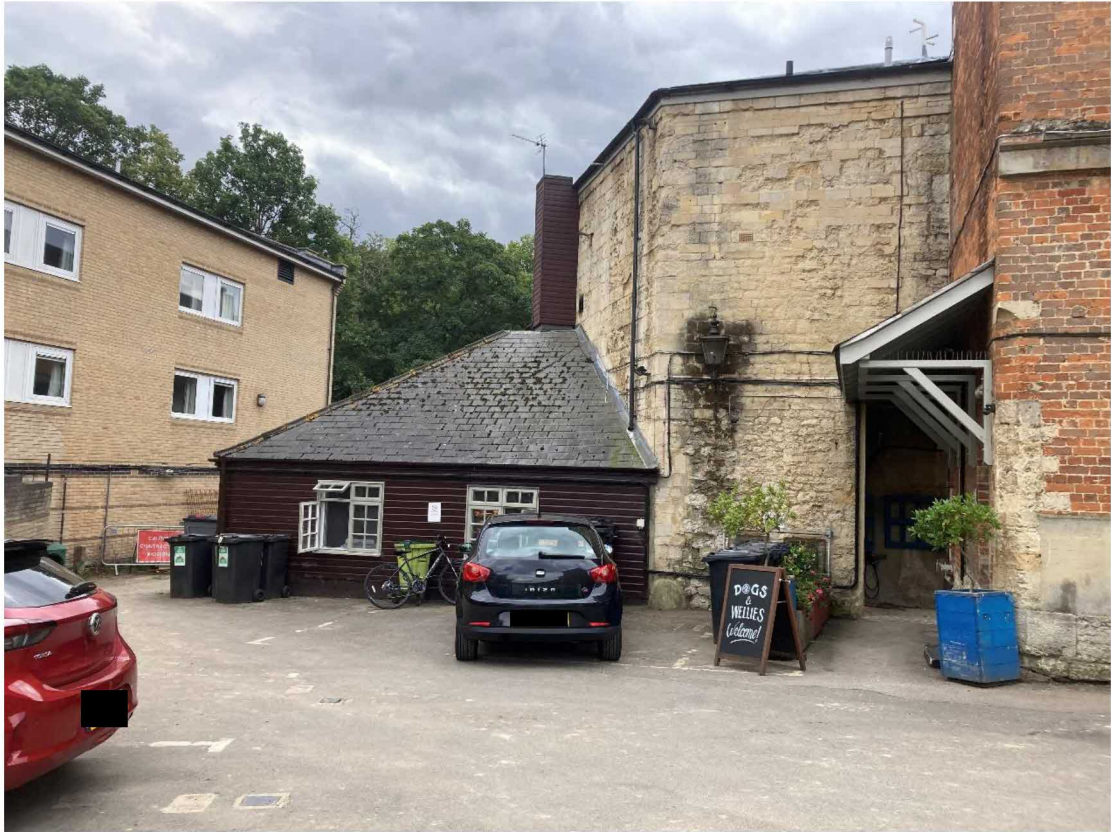
Above – Existing rear elevation of extended building and university halls of residence to left (east) of site, and original Wharf House to right (north) of site
