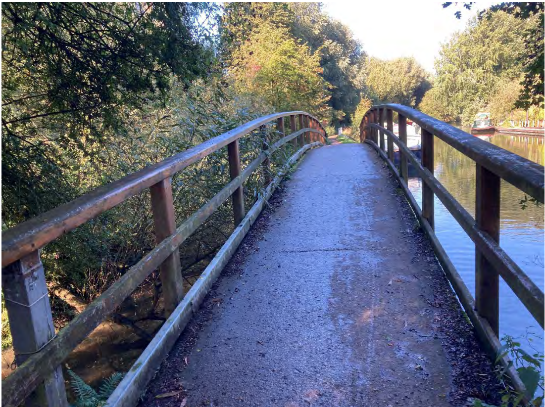
Photograph 12 – Footbridge over the Bulstake Stream
